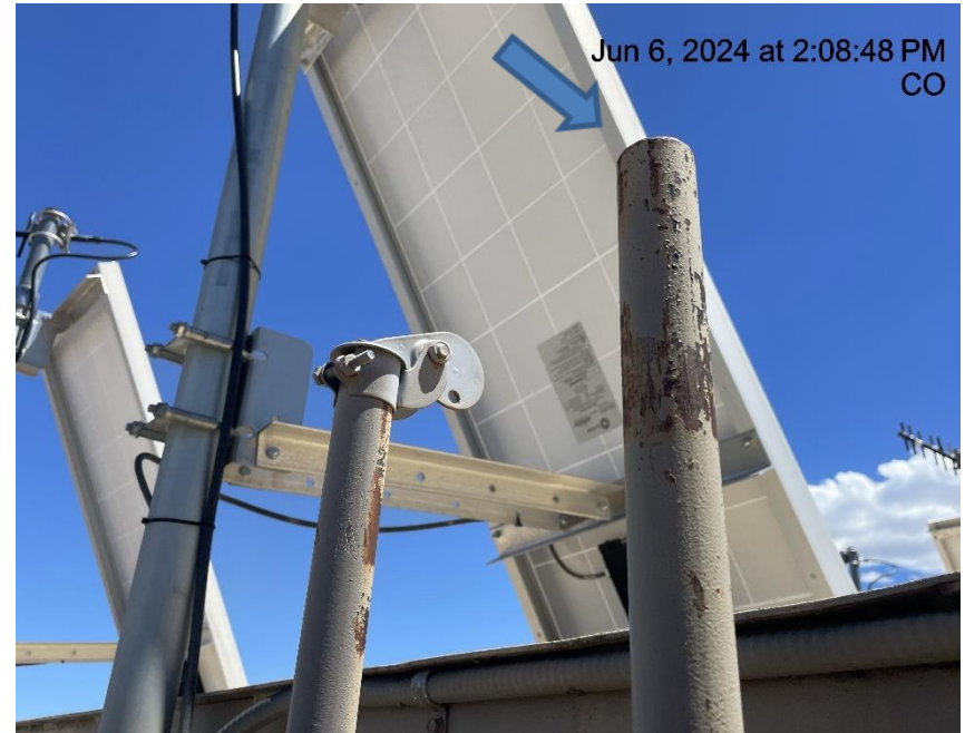
Photo # 55 PRV vent line does not comply with CECMC pressure safety device rules
