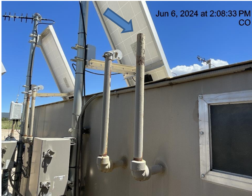
Photo # 54 PRV vent line does not comply with CECMC pressure safety device rules
