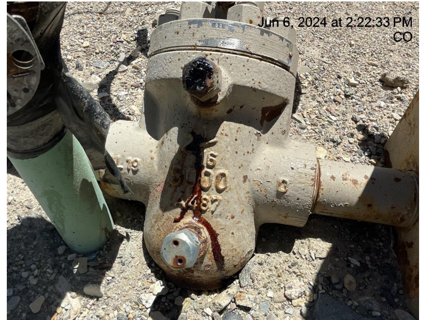
Photo # 53 Mechanical Condition - Possible leak on PA 332-6 wellhead casing valve
