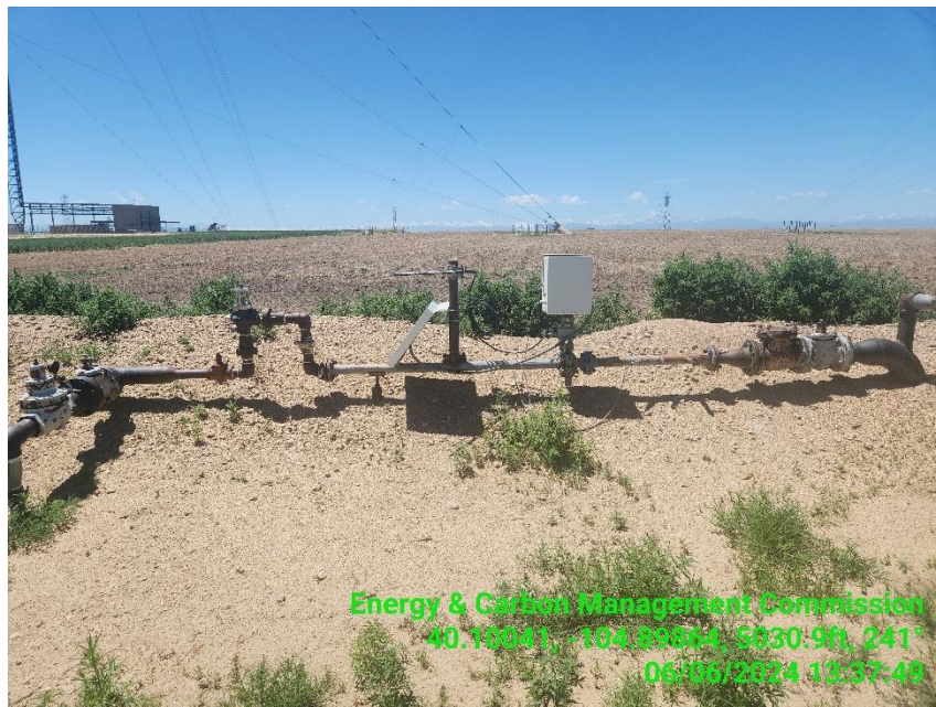
Photo 7 Gas Meter Run.
