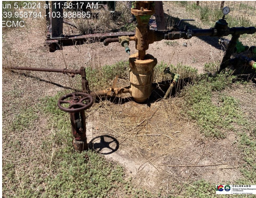
Pic 3 contaminated soil by wellhead
