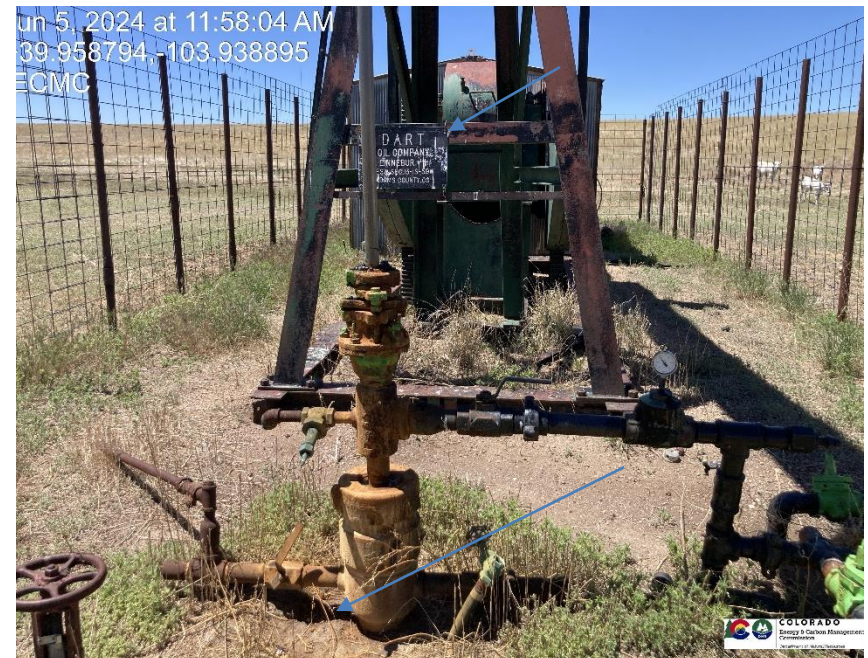
Pic 2 wellhead sign is inadequate. Wrong information.
