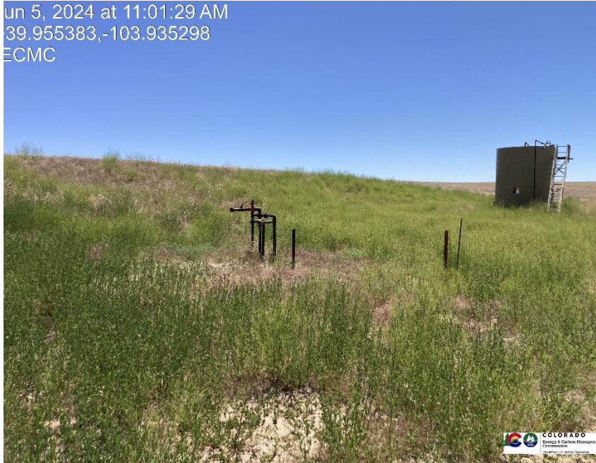
Pic 3 Weeds on location / Risers are not LOTO / Separator has been removed since previous inspection.
