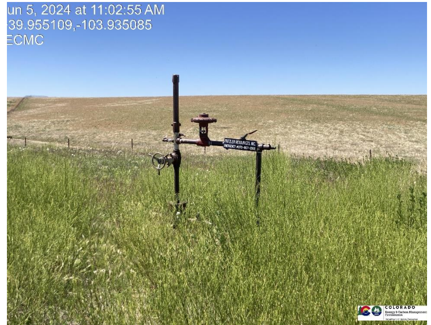
Pic 6 Wellhead sign is inadequate / weeds unmanaged
