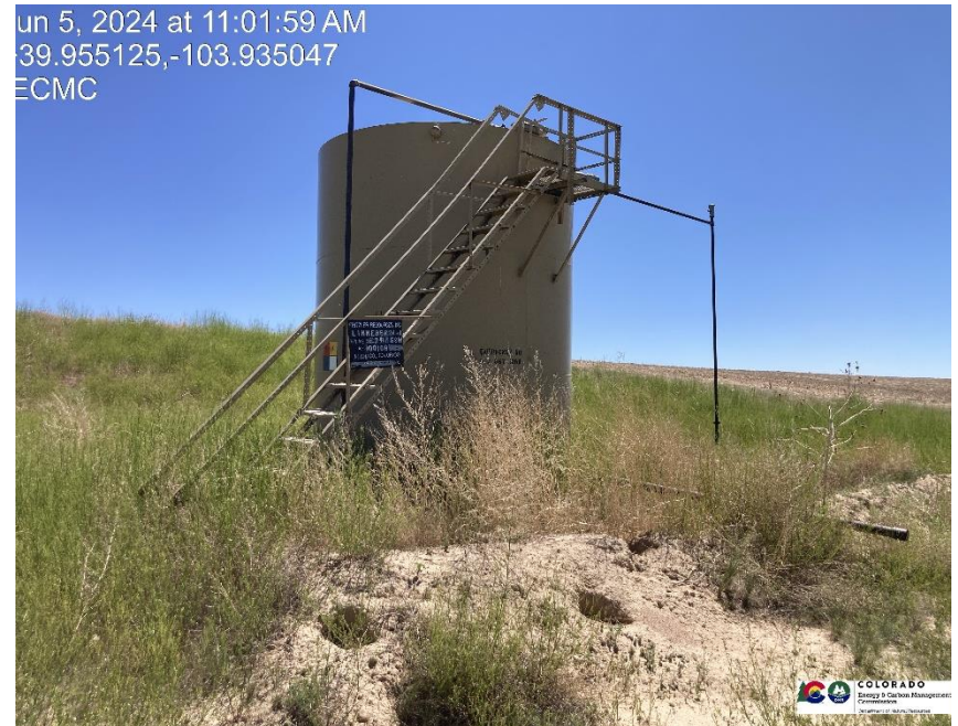
Pic 4 Berms need to be repaired around tank, weeds unmanaged.
