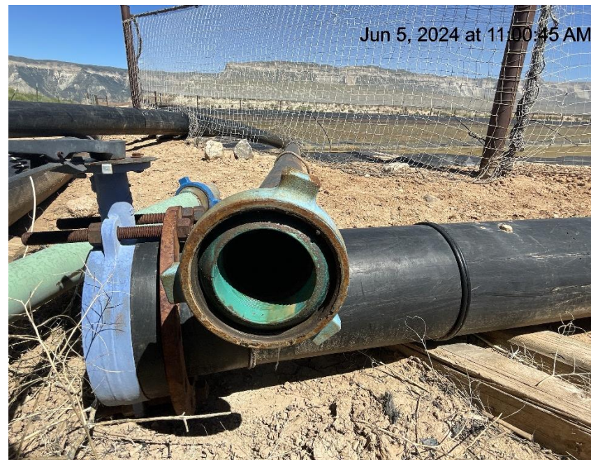
Photo # 9376 Open ended piping/wildlife hazard/available for entry by wildlife
