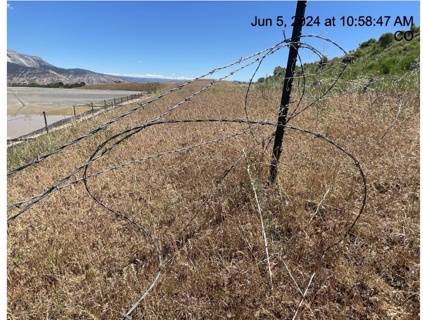
Photo # 9384 Barbed wire fence around location needs maintenance/wildlife hazard
