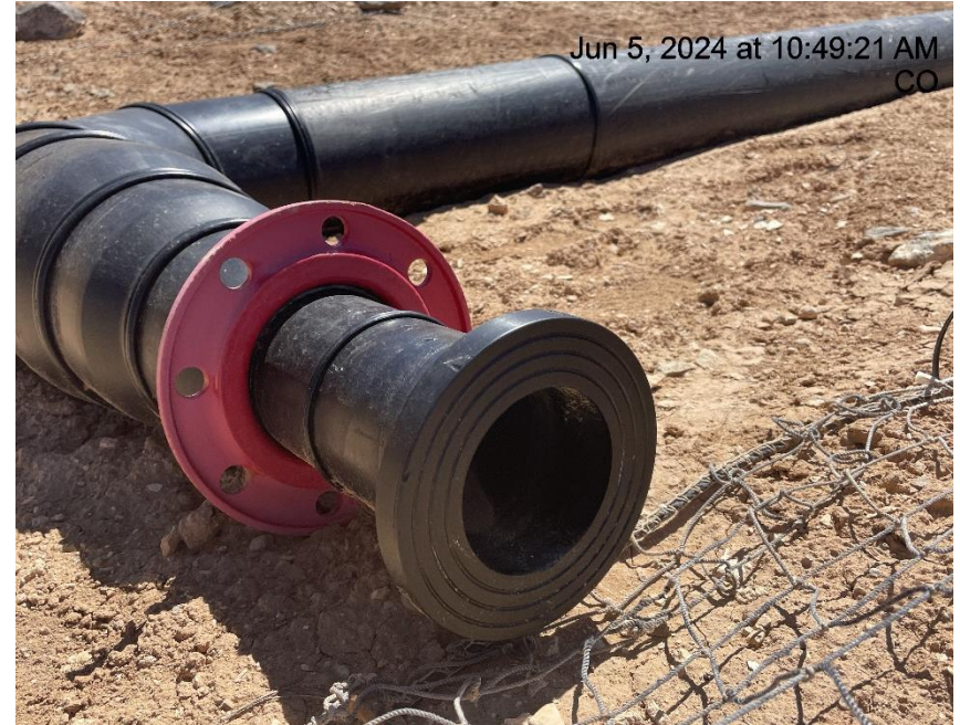
Photo # 9374 Open ended piping/wildlife hazard/available for entry by wildlife
