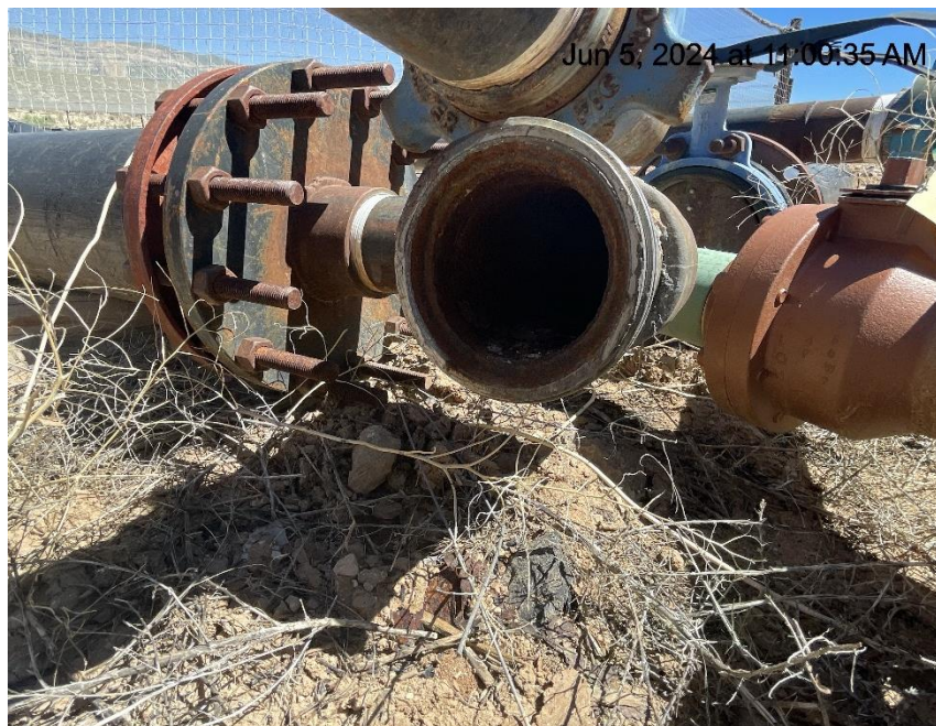
Photo # 9375 Open ended piping/wildlife hazard/available for entry by wildlife
