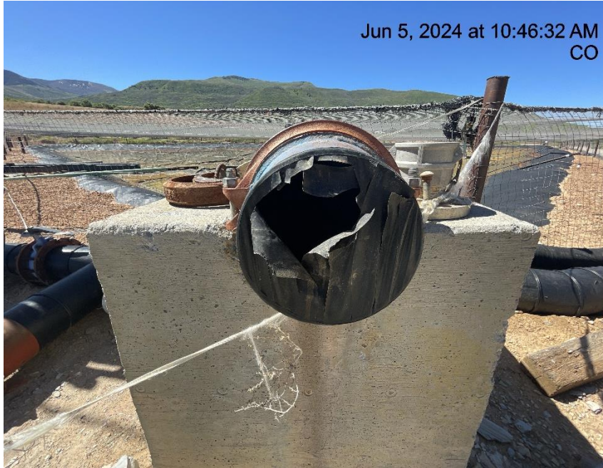
Photo # 9373 Open ended piping/wildlife hazard/available for entry by wildlife
