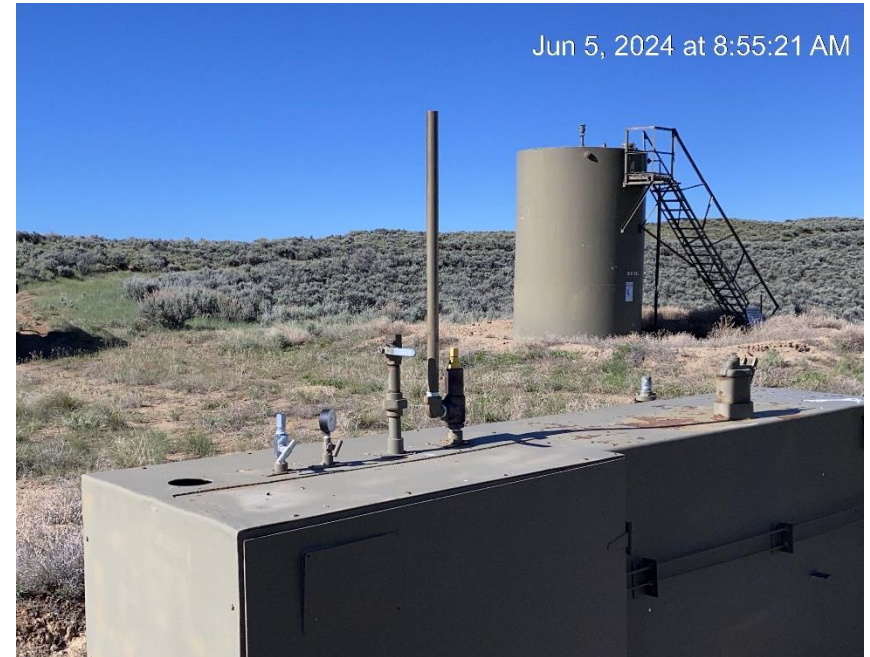
Unprotected relief riser
