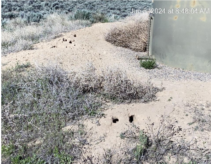
Insufficient tank berm
