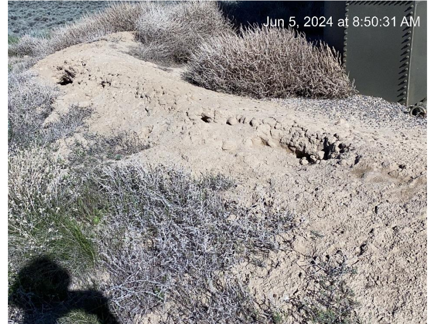
Insufficient tank berm
