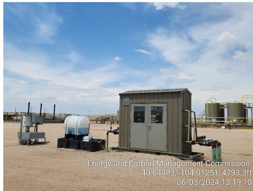
Photo 8 – Gas Lift Injection Meter House
