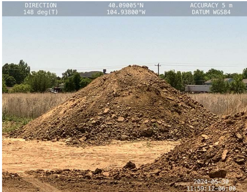
Photo 11 – Stockpiles unlined and unbermed
