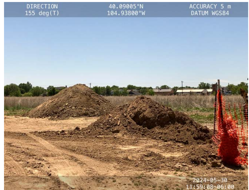
Photo 12 – Stockpiles unlined and unbermed
