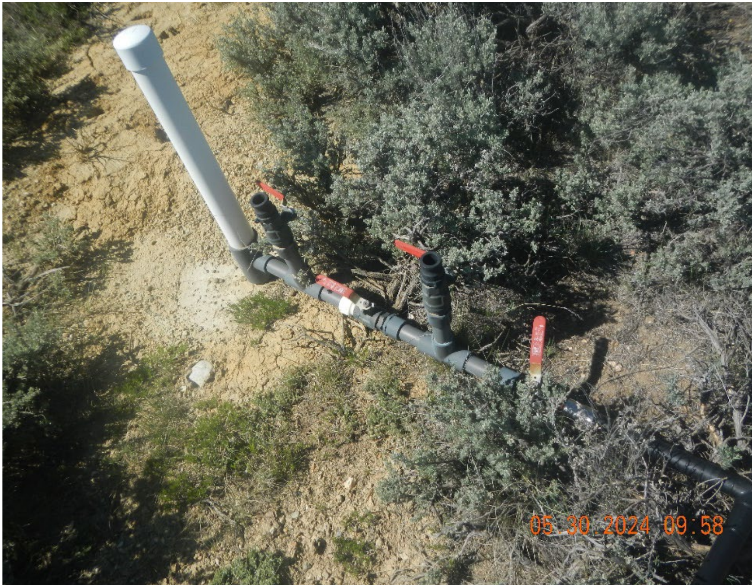
Photo #10 Sparge well and pipe. Note: the position of valve on right, it is throttled.
