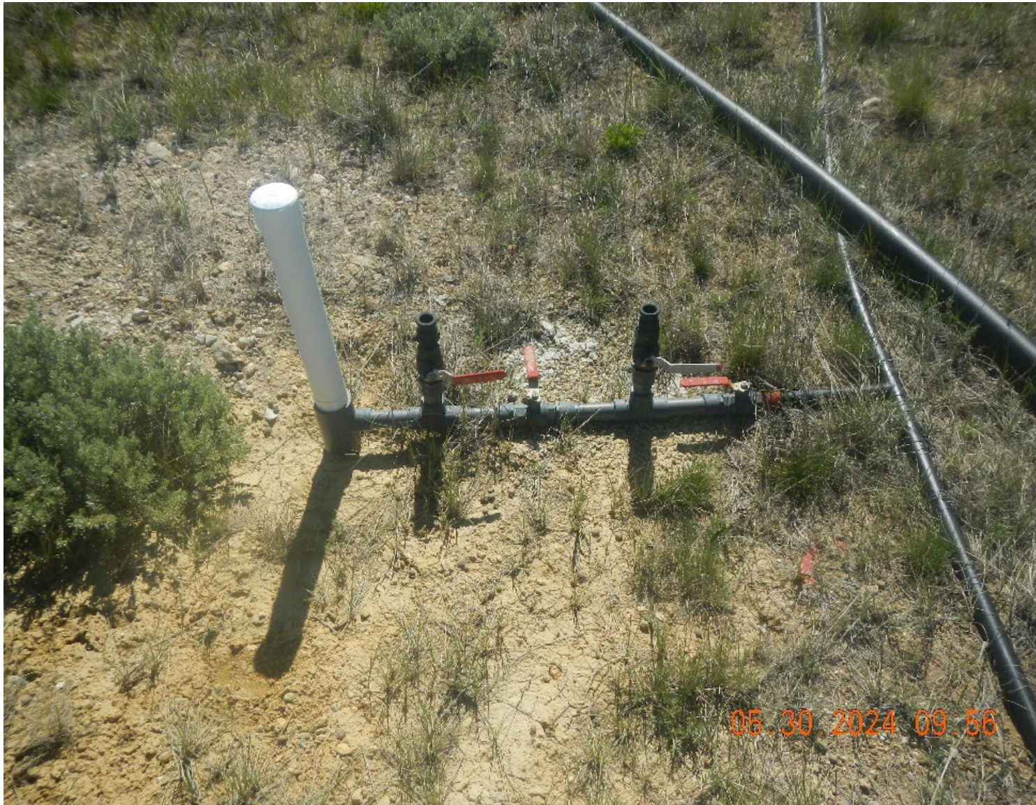
Photo #Sparge well and pipe. Note: the position of valve, it is throttled.
