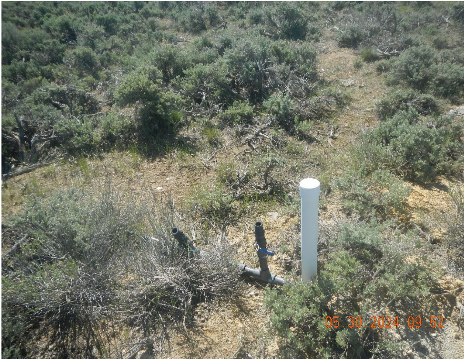
Photo #3 sparge piping.
