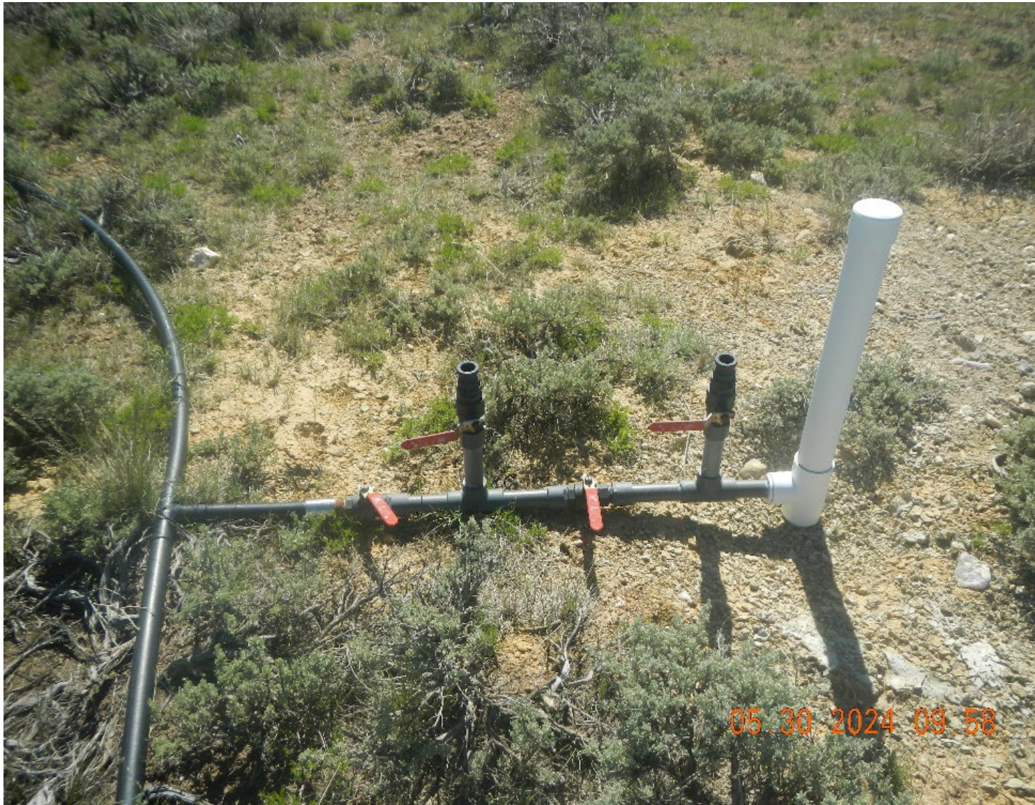
Photo #13 Sparge well and pipe. Note: the position of valves.
