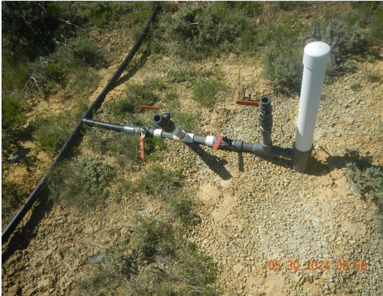
Photo #11 Sparge well and pipe. Both valves closed
