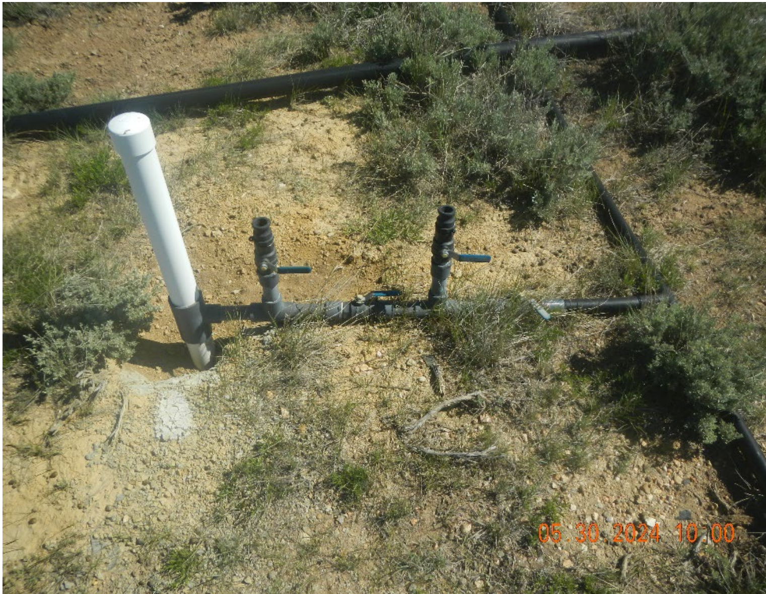
Photo #20 Sparge well and pipe. Note: the position of valve on right, it is throttled.
