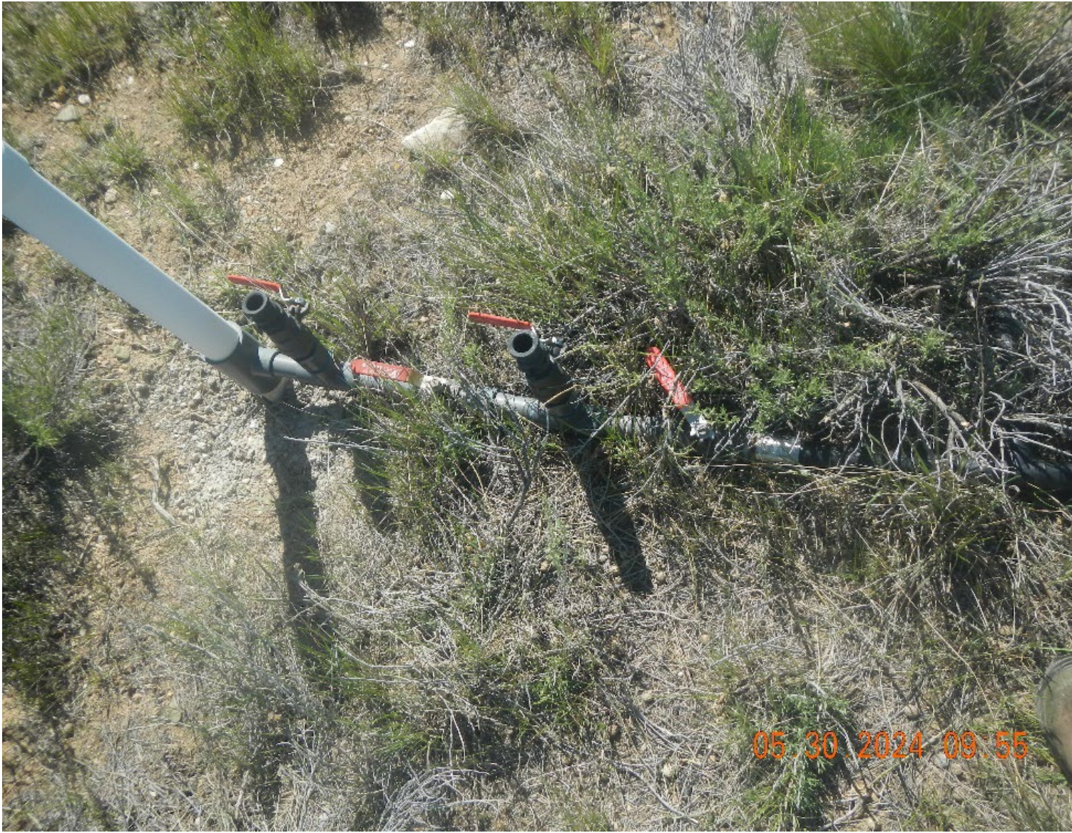
Photo #6 Sparge well and pipe. Note: the position of valve on right, it is throttled.
