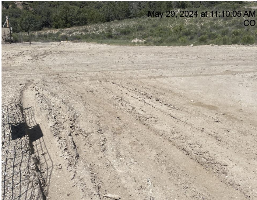
Photo # 8569 Lack of stabilization/compaction
