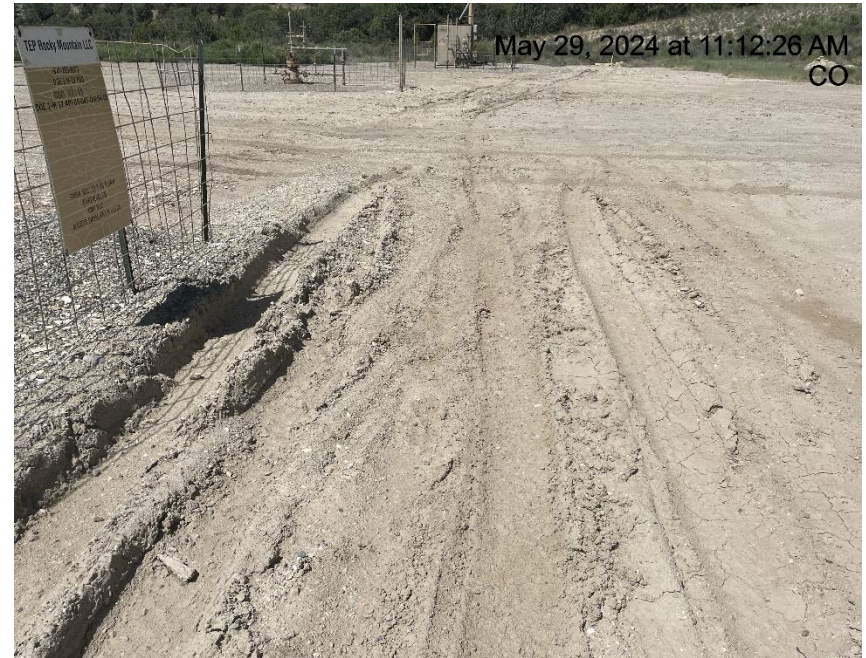
Photo # 8574 Lack of stabilization/compaction
