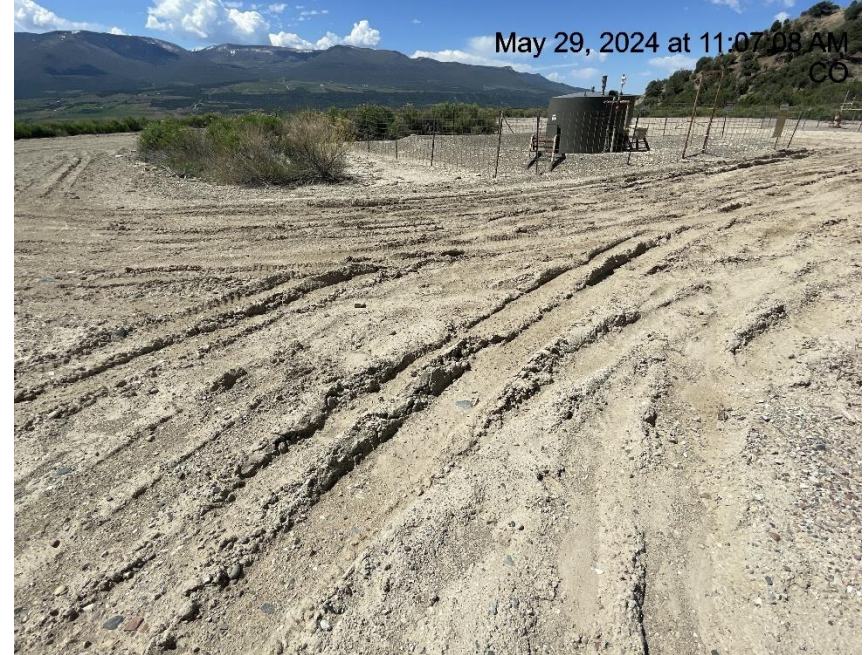
Photo # 8566 Lack of stabilization/compaction
