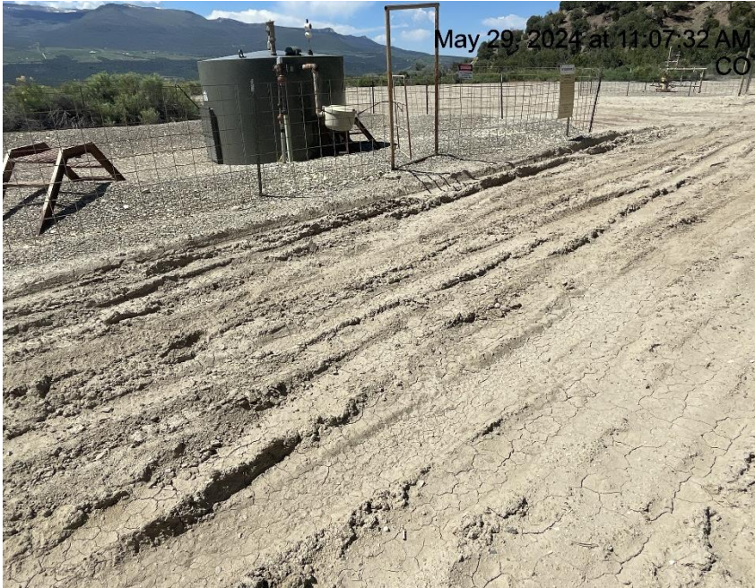
Photo # 8567 Lack of stabilization/compaction
