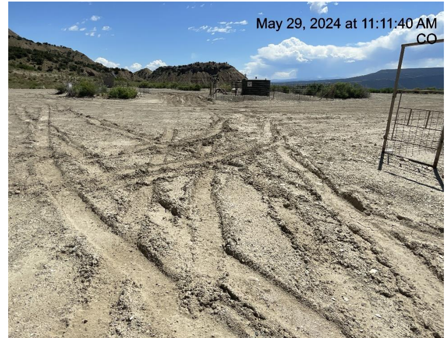
Photo # 8572 Lack of stabilization/compaction
