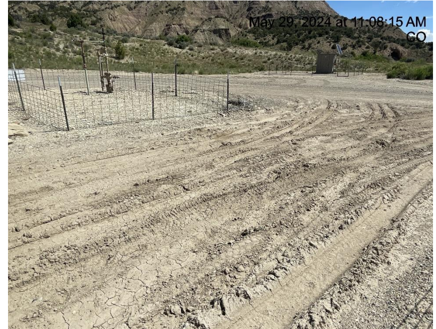
Photo # 8568 Lack of stabilization/compaction
