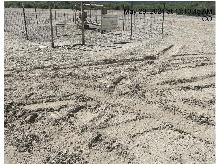
Photo # 8570 Lack of stabilization/compaction
