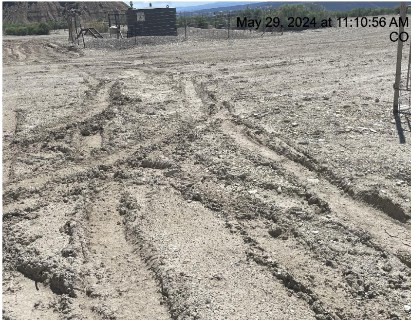
Photo # 8571 Lack of stabilization/compaction
