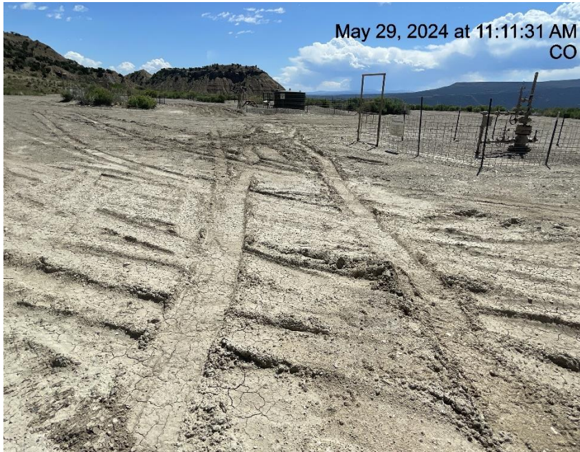
Photo # 8573 Lack of stabilization/compaction
