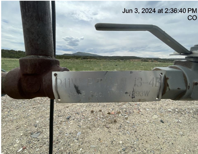
Photo # 9345 Wellhead sign lacks required information/sign does not comply with CECMC wellhead signage rules
