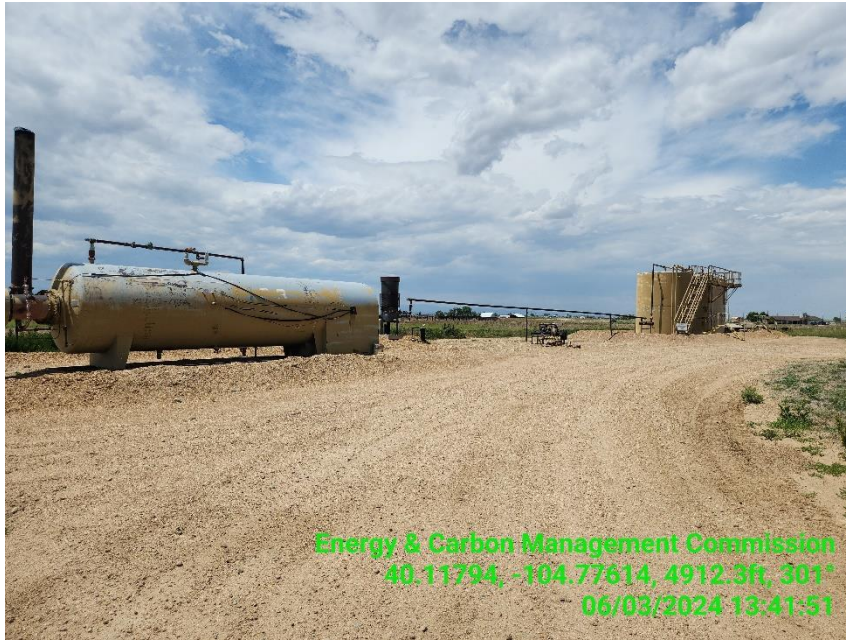
Photo 9 Tank battery location.
