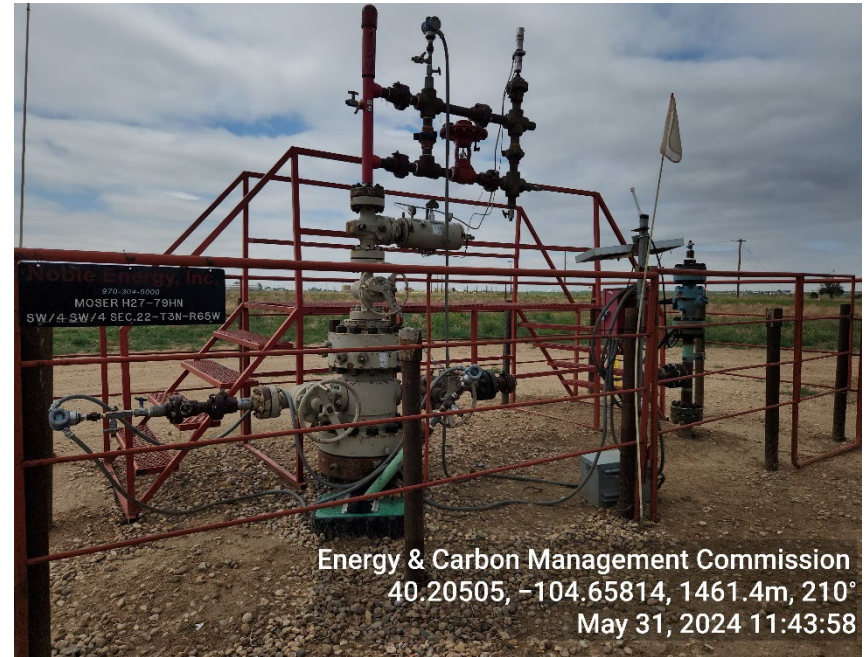
Photo 2: TA Wellhead
