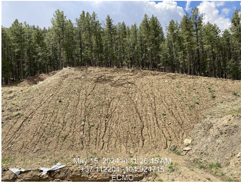
Photo 11 – Erosion Rills on cut slope
