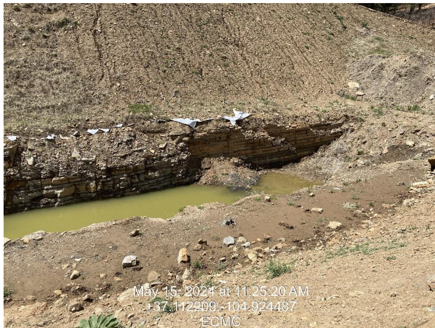
Photo 9 – Pit Facility ID 292612, fragments of pit liner let around edge of trench.
