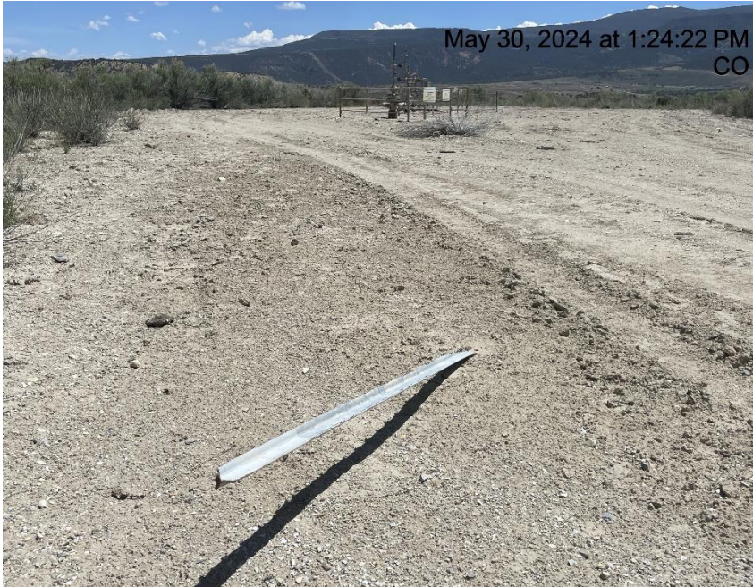
Photo # 9039 Improperly marked deadman
