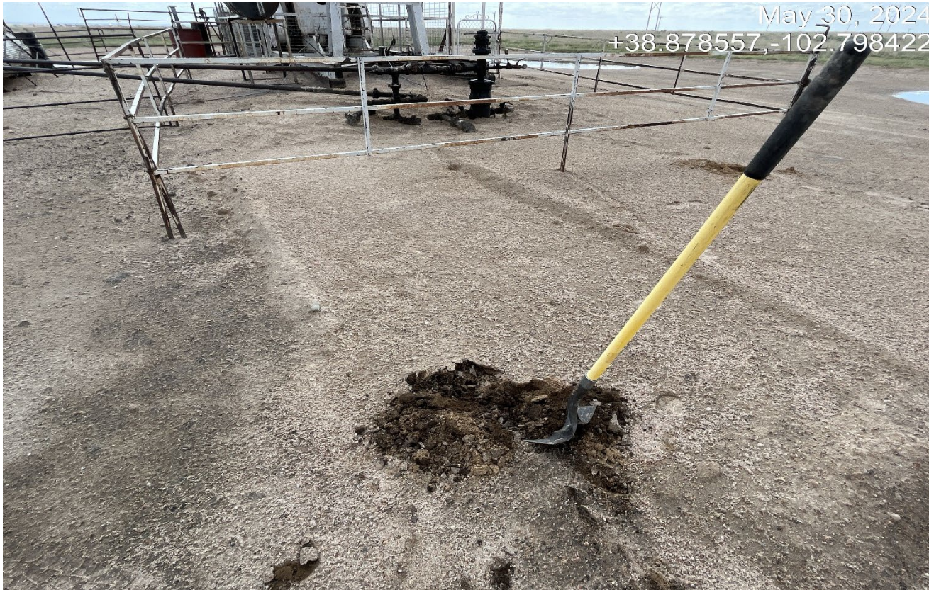
Photo 4. It appears there was sand spread on top of the spill which was not cleaned up per the rules.
