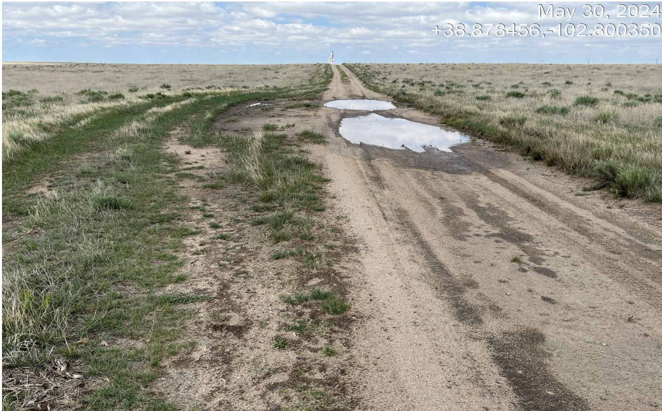
Photo 8. Facing west along the access road. Vehicles are causing unnecessary disturbance driving outside of the access road due to stormwater pooling on the road. The access road must be maintained and shall not drive outside of the access road boundary.
