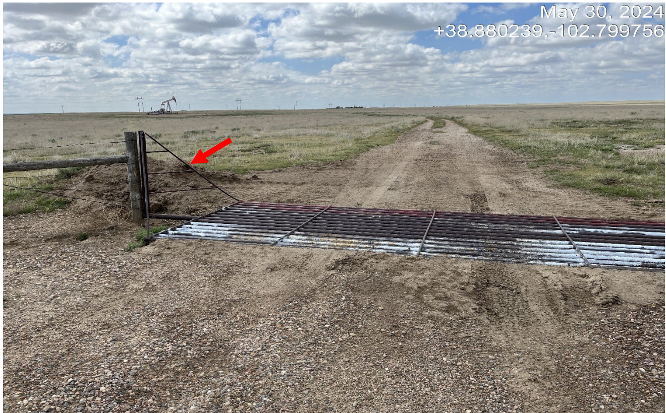
Photo 1. The cattleguard at the beginning of the access road has been cleaned out but the material was set to the side and needs to be removed.
