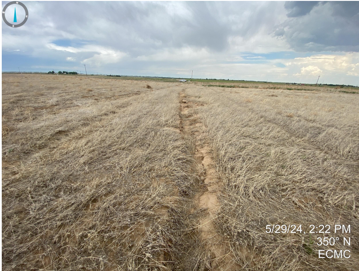
Photo 8. Erosion degradation occurring along the former access road; facing north.
