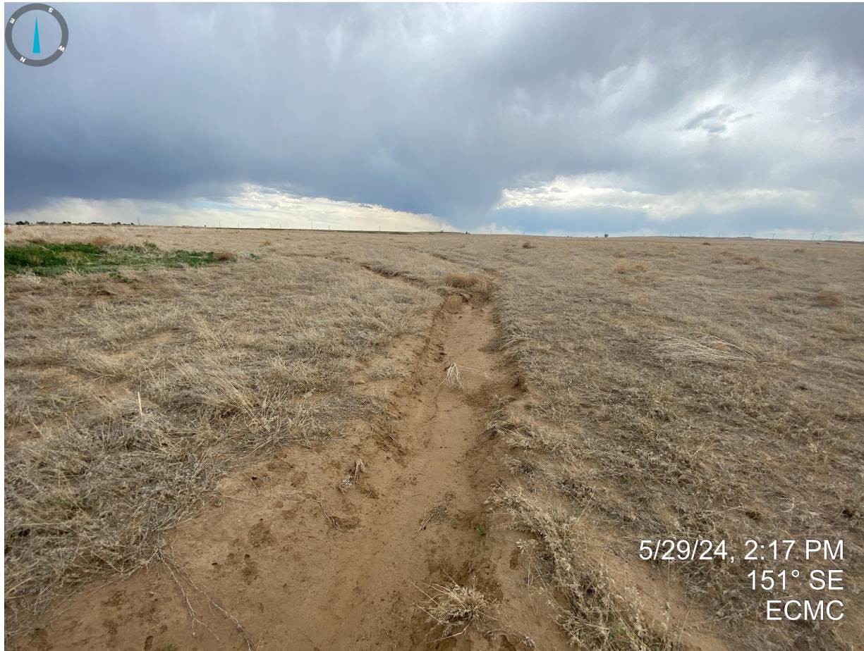
Photo 1. Erosion degradation occurring along the former access road; facing southeast towards the former location.
