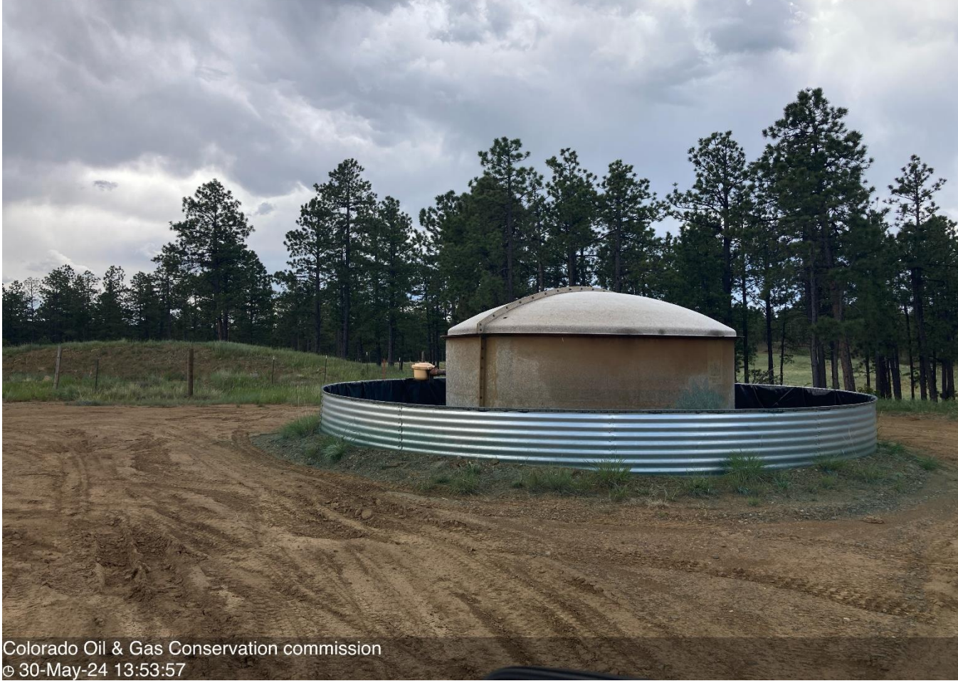
PHOTO 5: USED OIL TANK BATTERY
