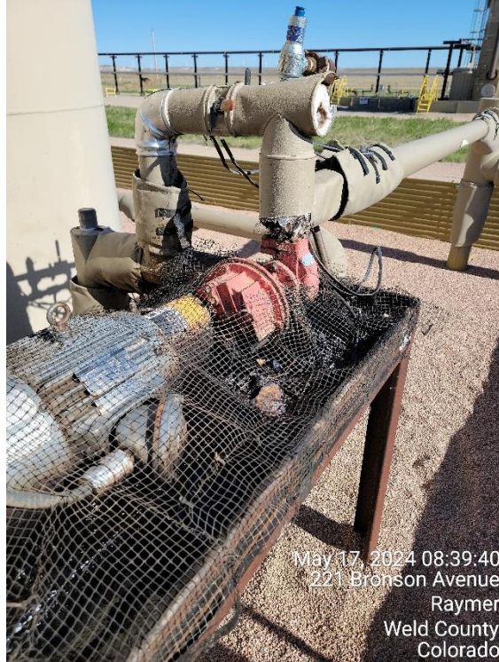
Razor 22D – Wildlife Protection Netting Has Been Restored With Hydrocarbons Below Netting At Recycle Pump & Not Accessible To Wildlife
