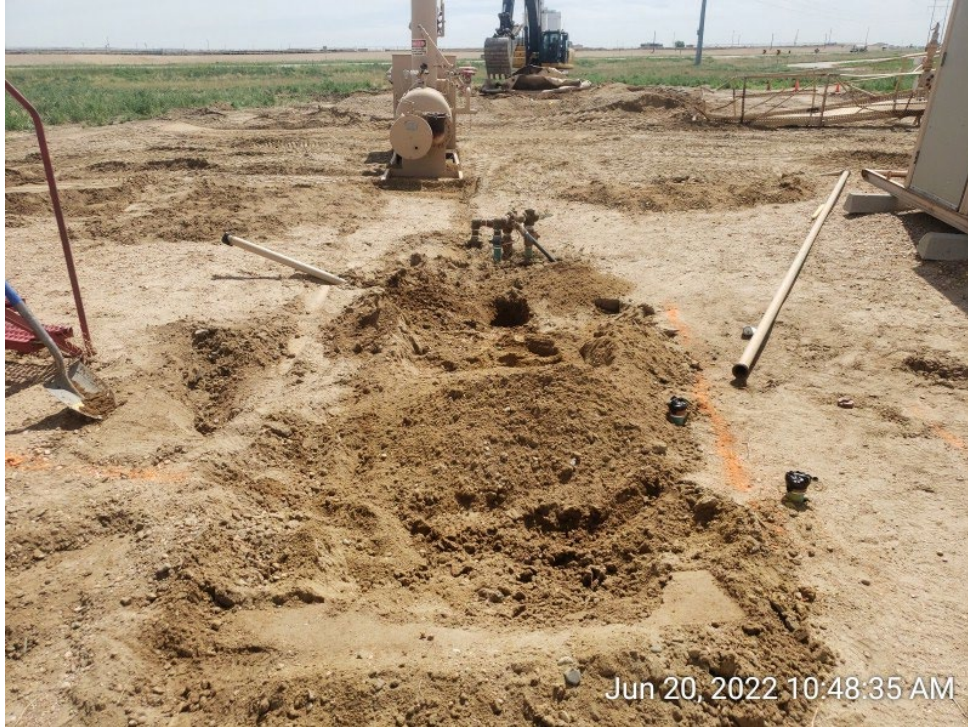
#7B - UPRC-65N64W 23SESW – Separator – SEP01@6.0” – No Impacts Noted – PID 0.3ppm – Sample Submitted for Lab Analysis – Facing East
