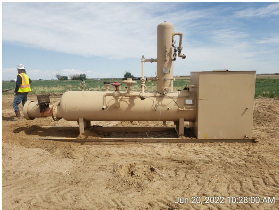
#7A - UPRC-65N64W 23SESW – Separator – Good Condition – Little to No Corrosion – Facing North
