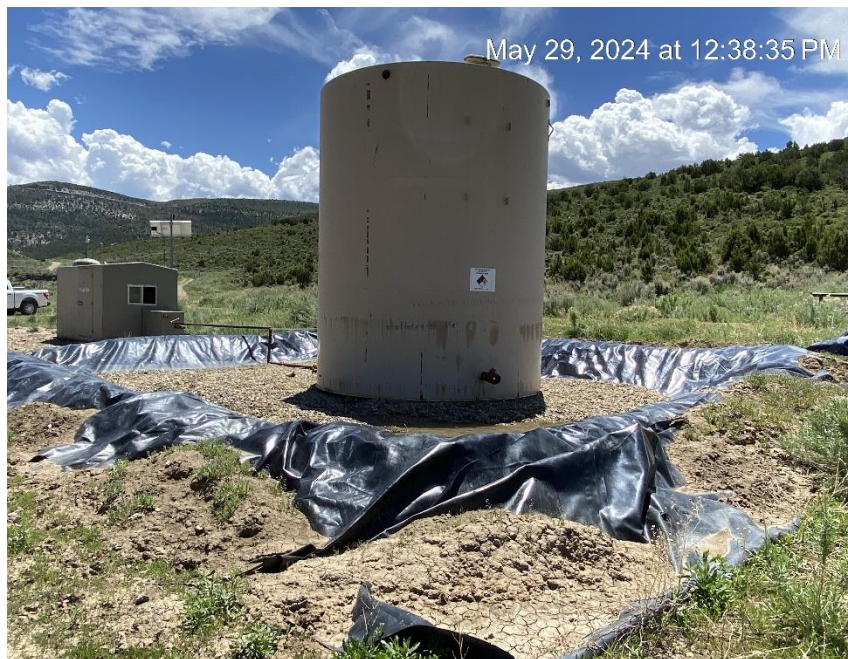
Containment undersize
