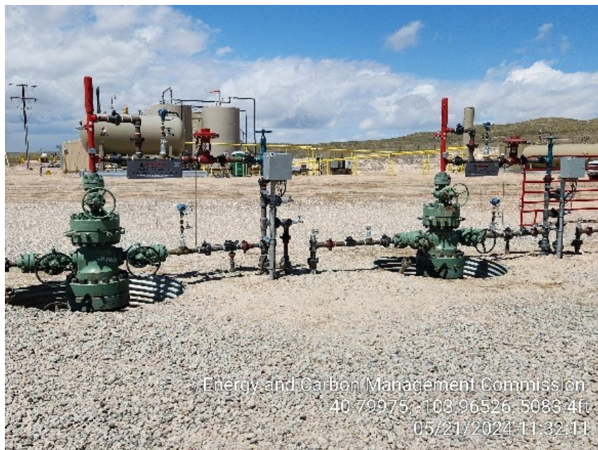
Photo 7 – Wellheads – Cellars NOT back filled in
