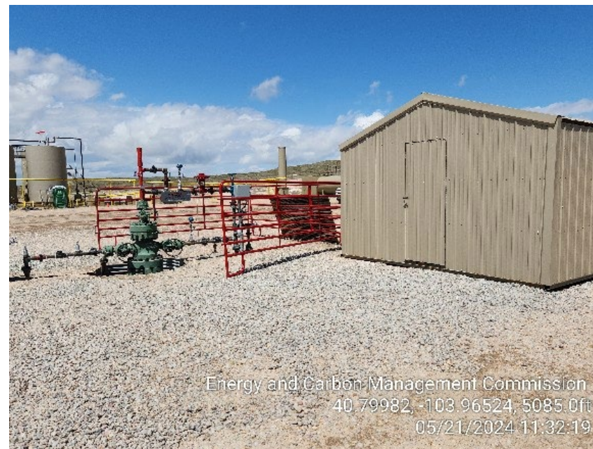
Photo 8 – Wellhead and Gas Lift Injection Meter House – Cellars NOT back filled in
