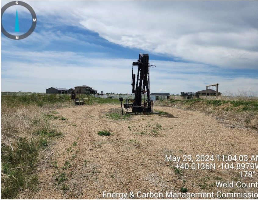
Photo 1 well head and equipment
