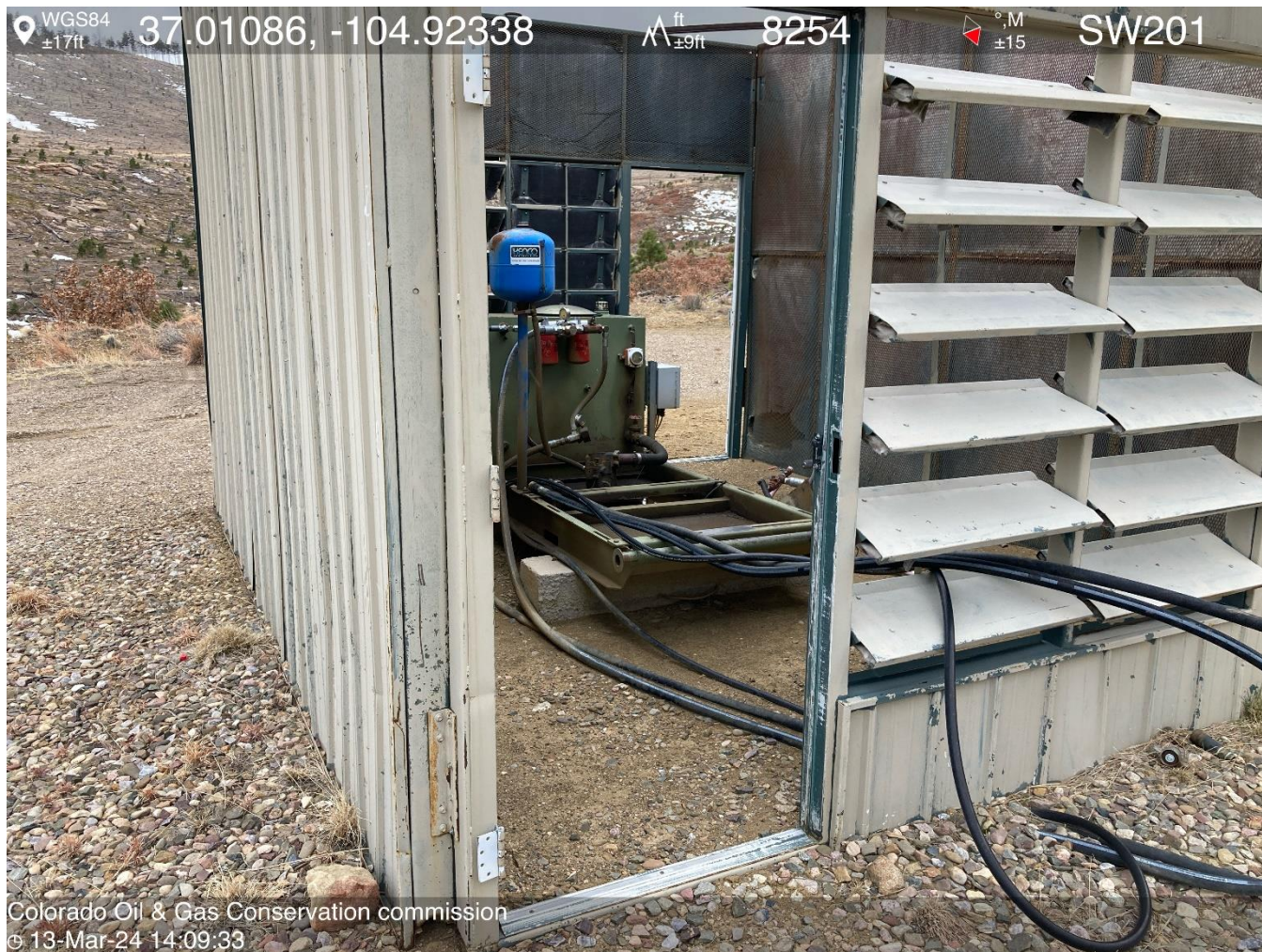
PHOTO 4: ENGINE SKID AND SOUND WALLS ARE UNUSED EQUIPEMT AND SHOULD BE PUT BACK IN WORKING ORDER OR REMOVED FROM LOCATION.
