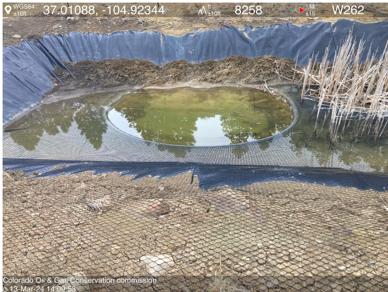
PHOTO 5: NETTING IS TORN AND PART OF IT IS BELOW WATER. REPAIR NETTING.
