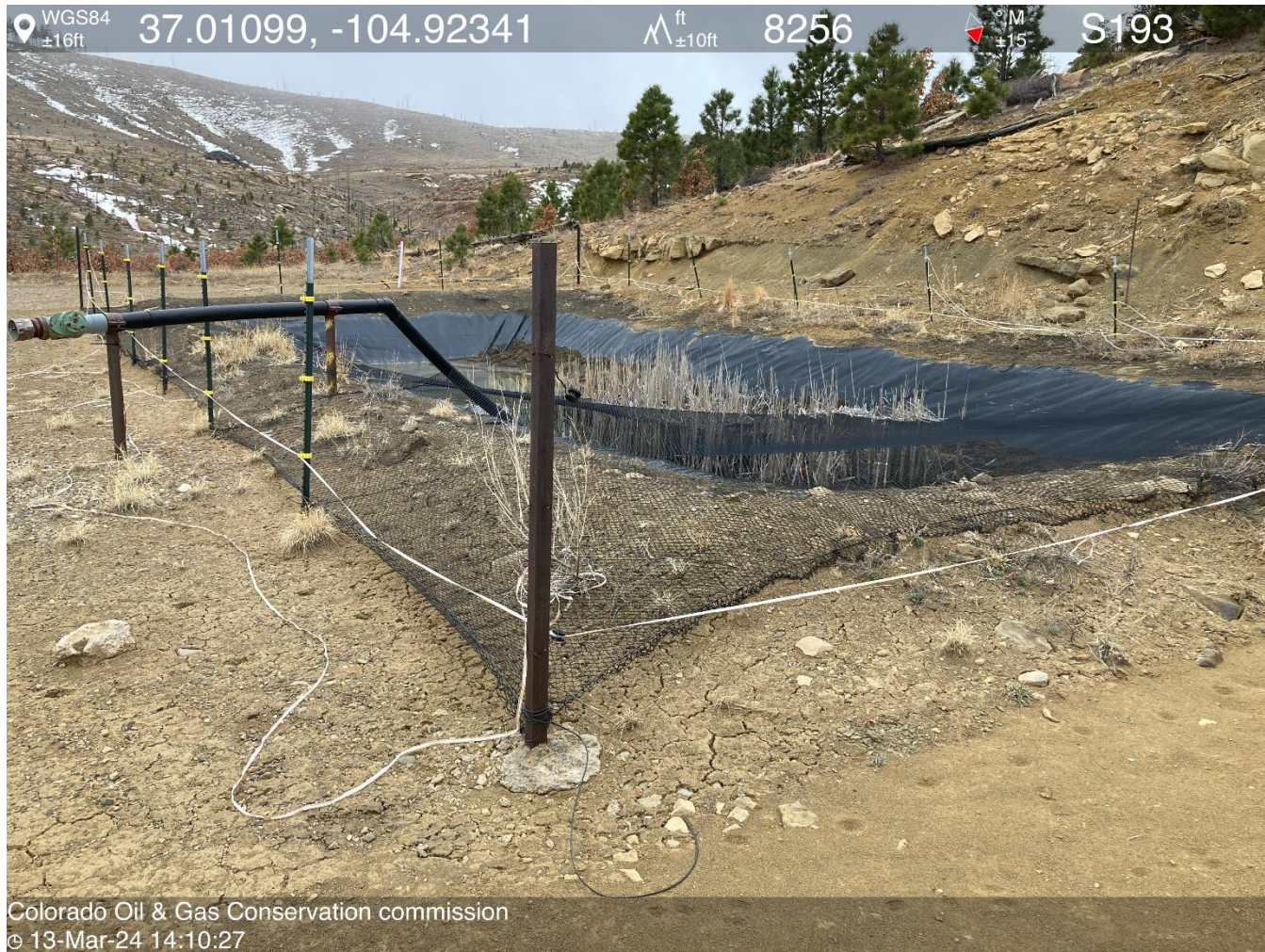
PHOTO 6: FENCING AROUND LINED PIT IS DOWN. REPAIR FENCE.
