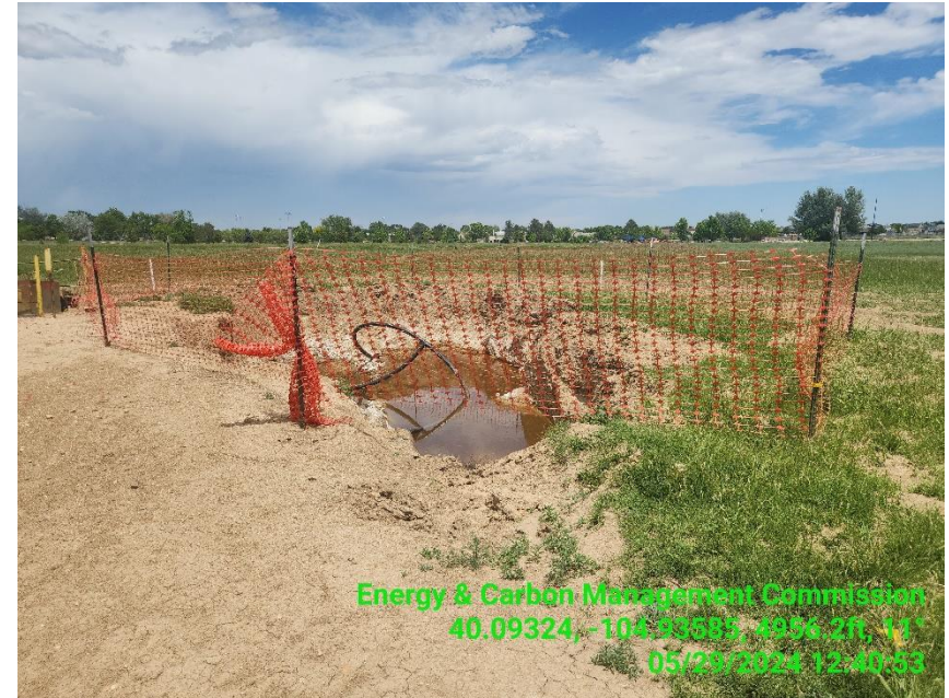
Photo 6 Unfinished Flow line/pipeline repair excavation, with pooled standing water.
