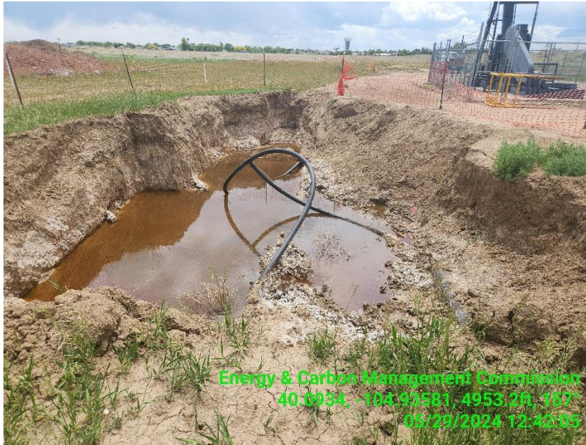
Photo 7 Unfinished Flow line/pipeline repair excavation, with pooled standing water.
