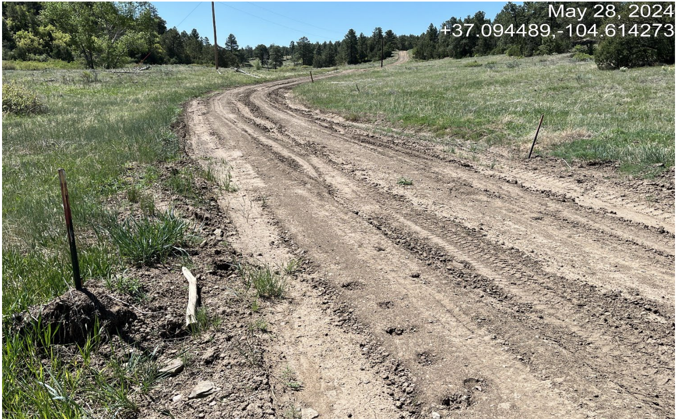
Photo 1. Facing south along the access road. There is vehicle rutting along the road that needs to be repaired.
