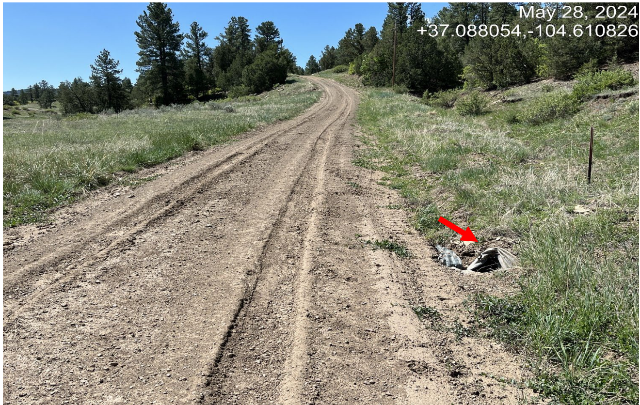
Photo 2. Facing south along the access road. This culvert is damaged and the outlet has filled in with sediment.
