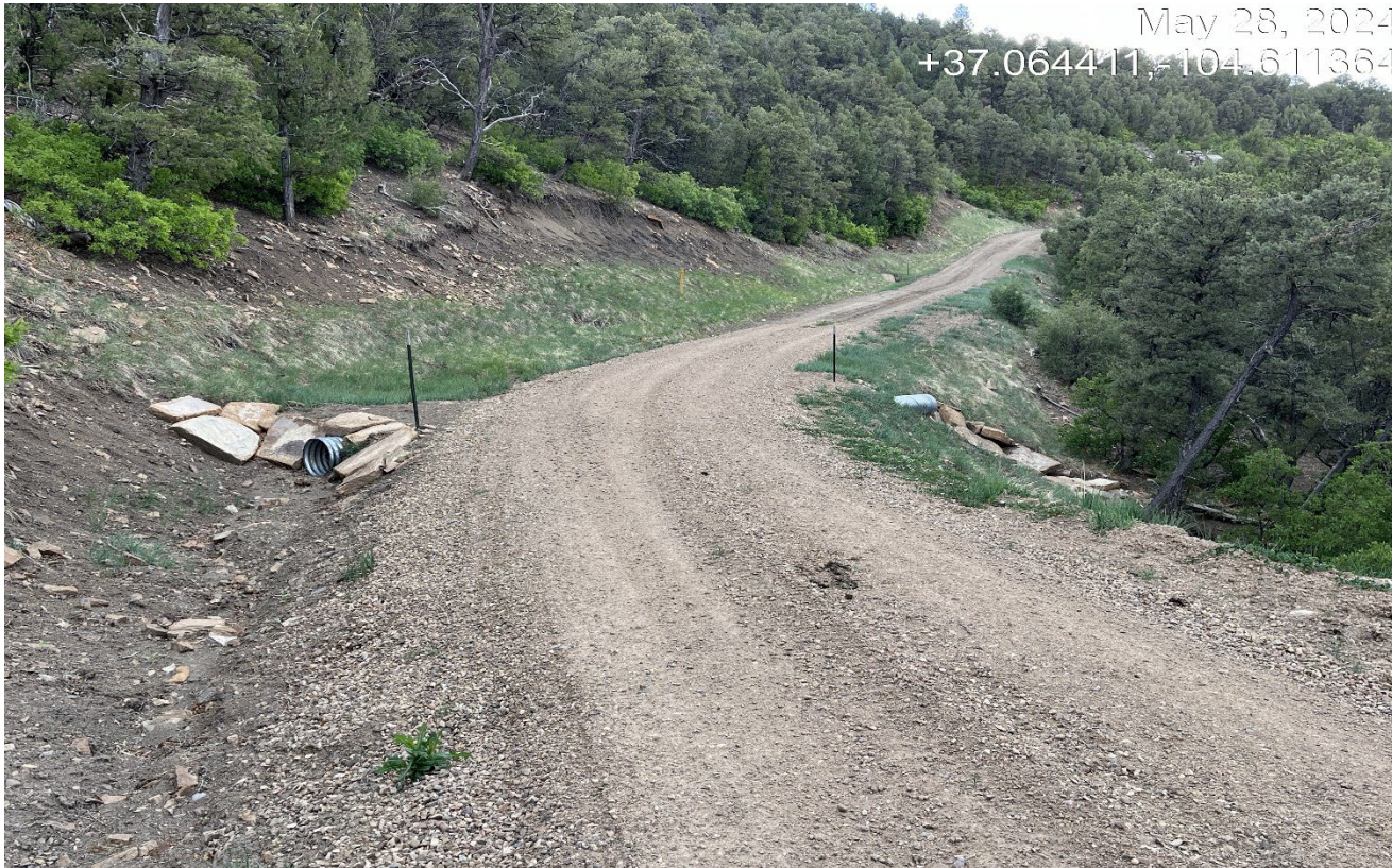
Photo 2. Facing south along the access road. A new culvert was installed with outlet protection.
