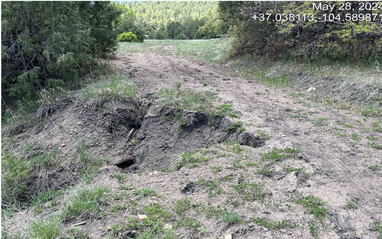
Photo 1. Facing south along the pre-existing access road. This area has washed out and needs to be repaired.
