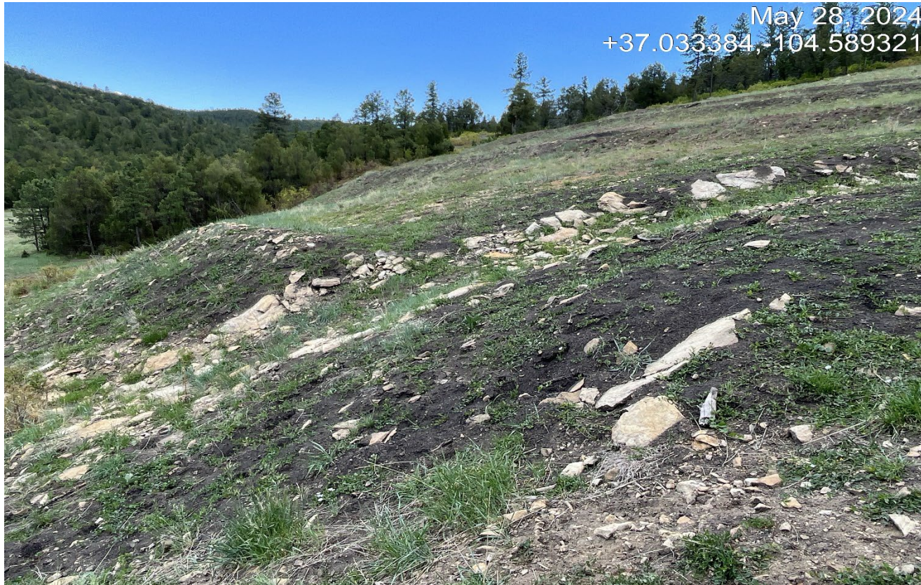
Photo 13. Facing south toward the lower portion of the location. The large berms are filled in with sediment and are increasing the steepness of the slope toward the bottom. Regrading the lower portion of the location may be beneficial as the vegetation is not progressing.
