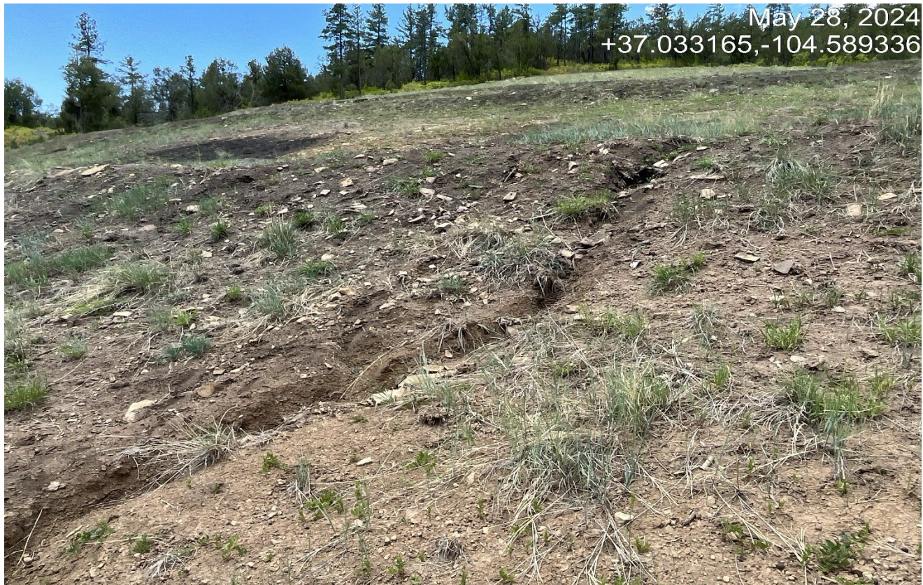
Photo 6. Facing southwest. The berms along the slope have filled in and eroded
