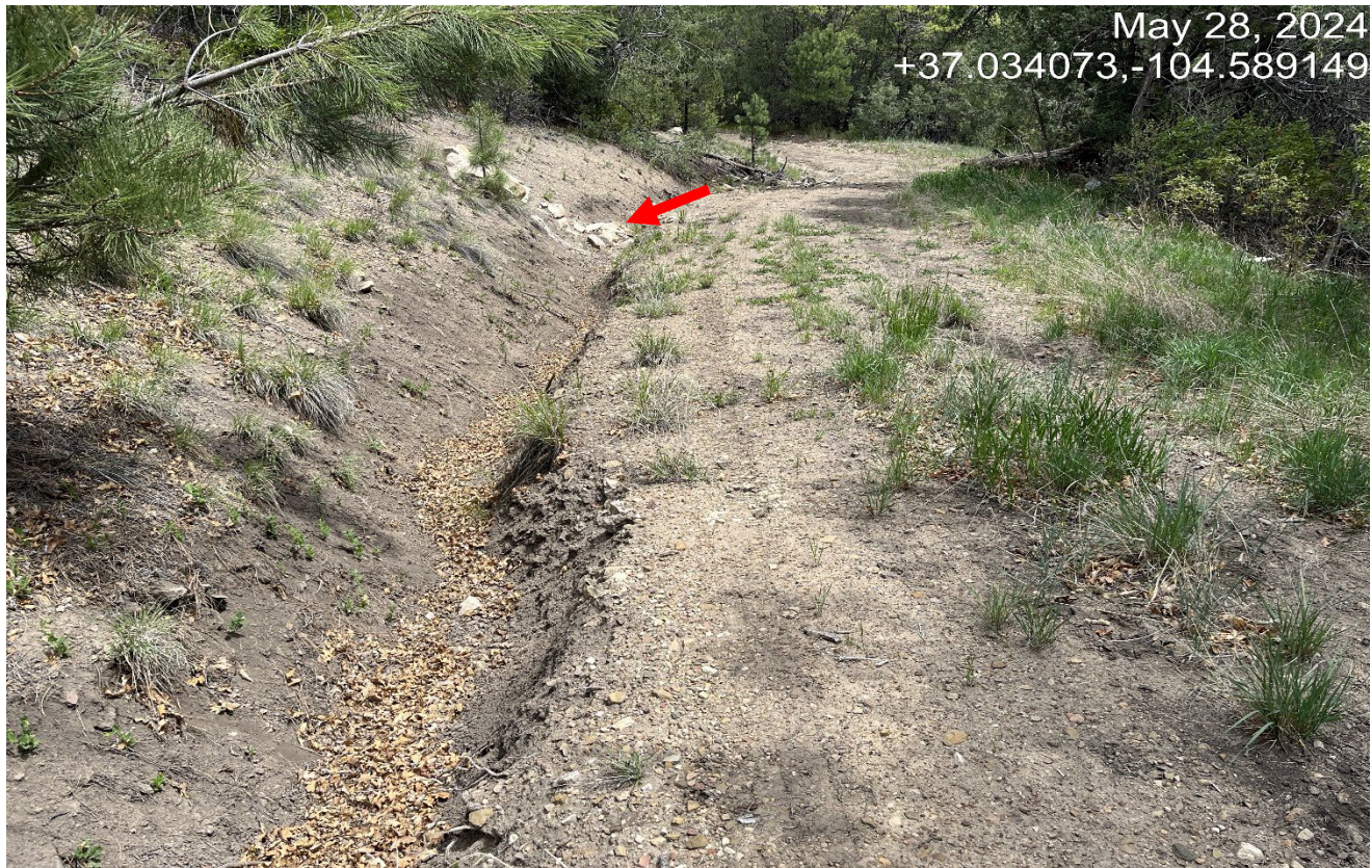
Photo 3. Facing back northeast down the road. Stormwater from the location is directed down the roadside with insufficient BMP's. There is a rock check dam at red arrow that has filled in with sediment.
