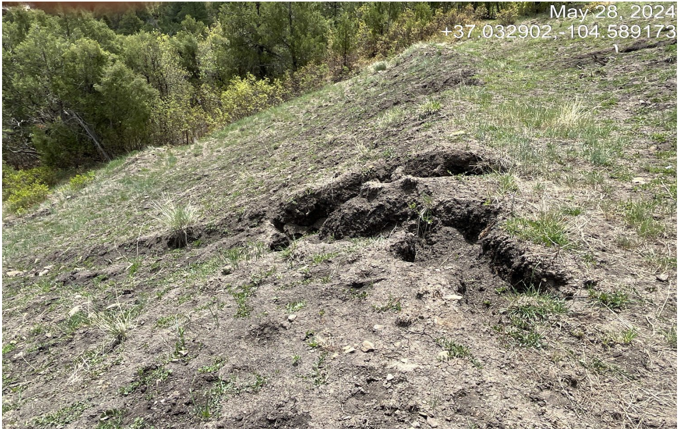
Photo 7. There are several areas where erosion has occurred along the slope where berms have concentrated stormwater flow..
