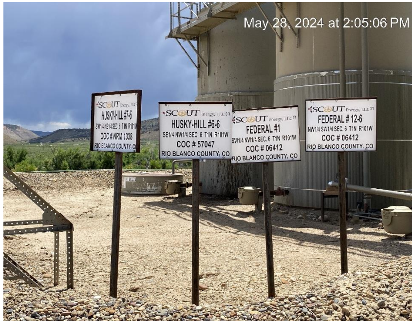
Tank battery signs missing required information
