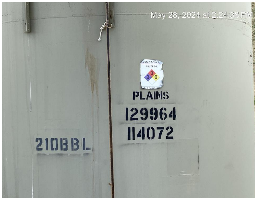
Replace damaged, faded and illegible labels
