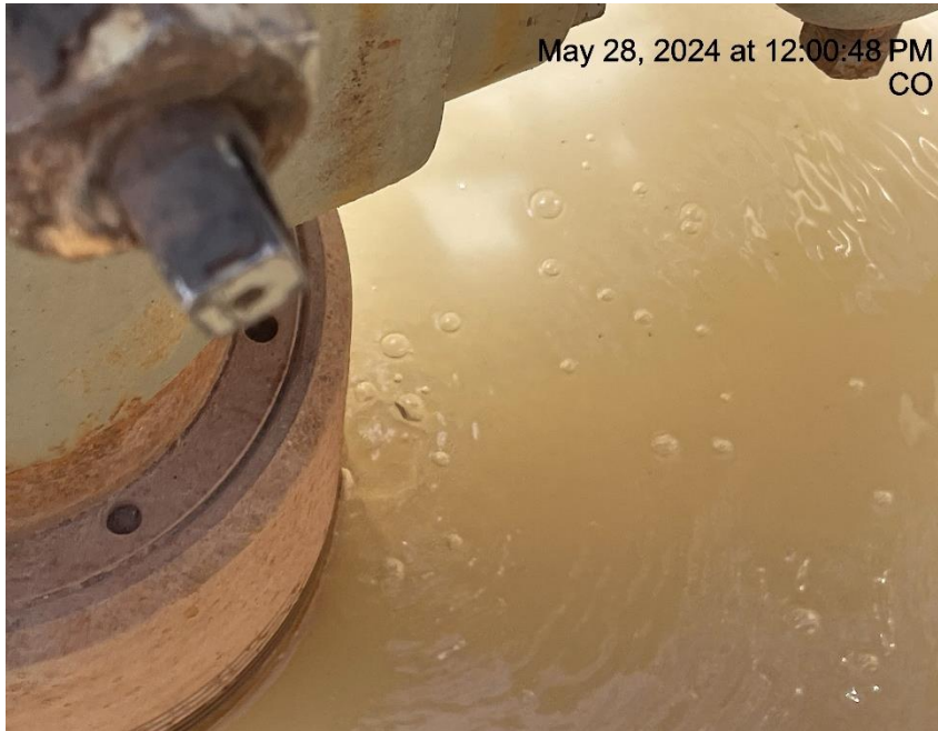
Photo # 8449 Possible wellhead leak/gas bubbling up around wellhead through water in cellar
