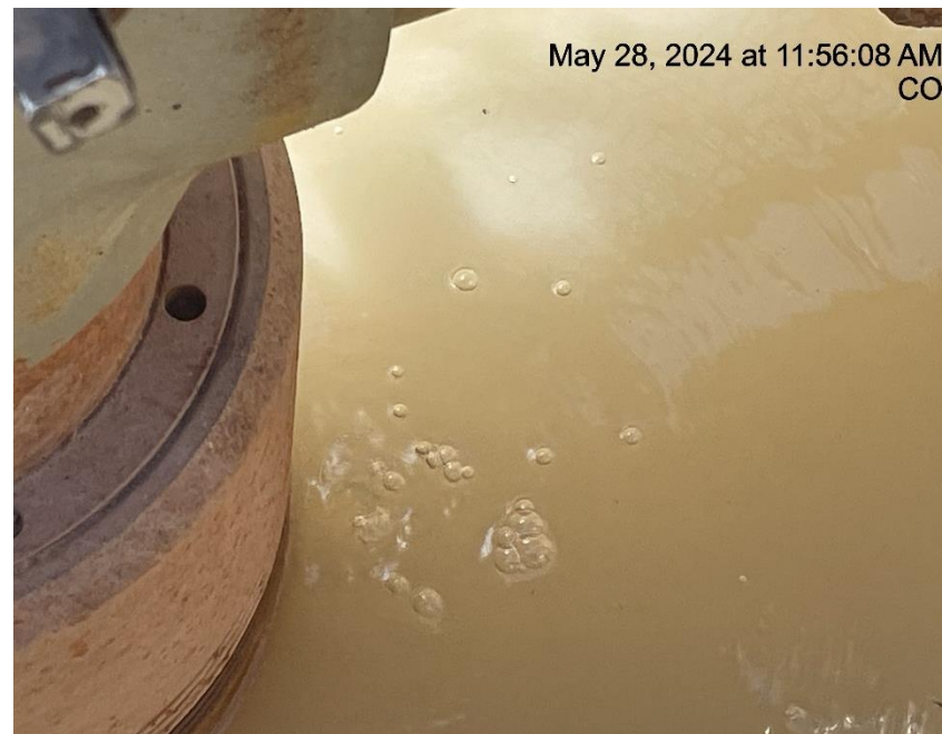
Photo # 8448 Possible wellhead leak/gas bubbling up around wellhead through water in cellar
