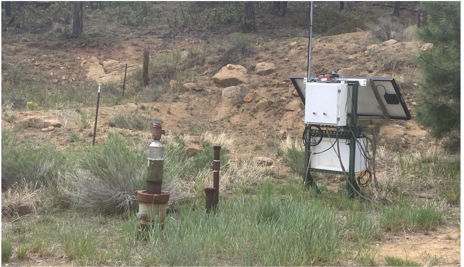
PHOTO 3: V WELLHEAD AND EQUIPMENT
