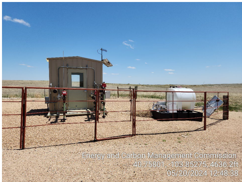
Photo 1 – Gas Lift Injection Meters
