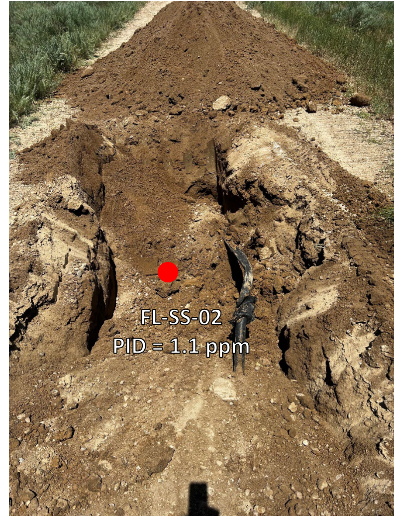
Looking north at bellhole/cut point for removal
