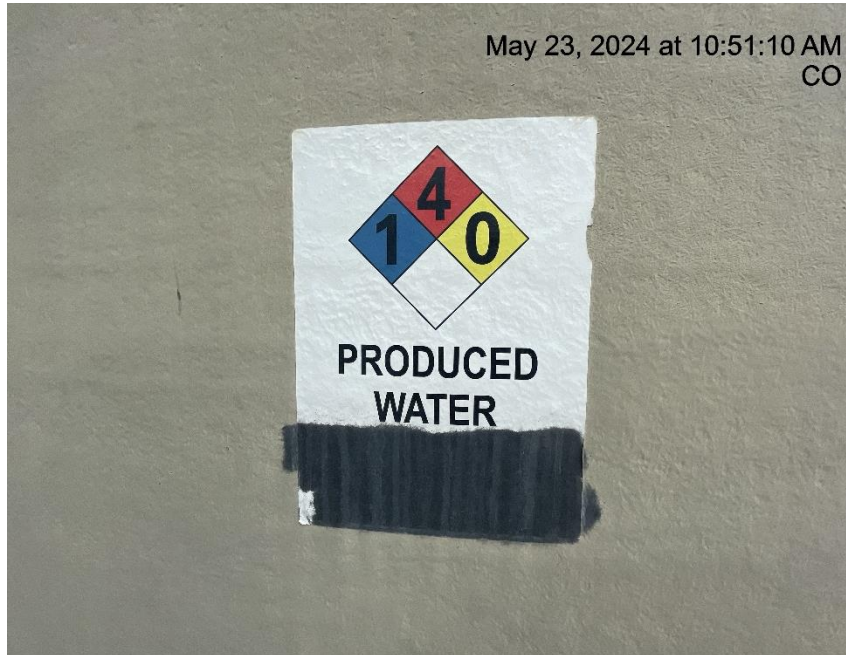
Photo # 8189 Tank label missing required information/does not comply with CECMC rules
