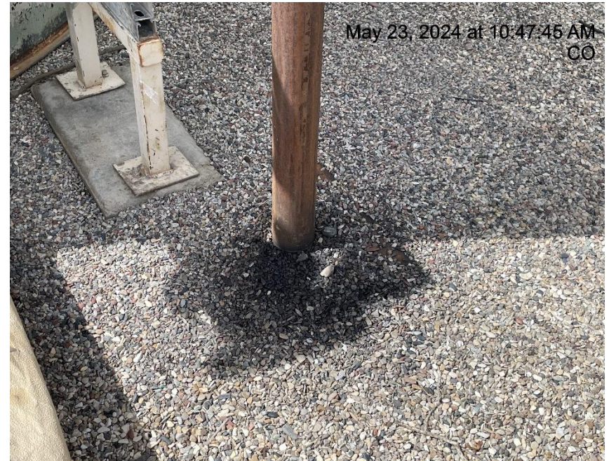
Photo # 8200 Staining in secondary containment
