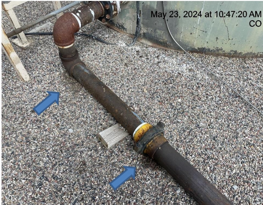
Photo # 8201 Staining in secondary containment
