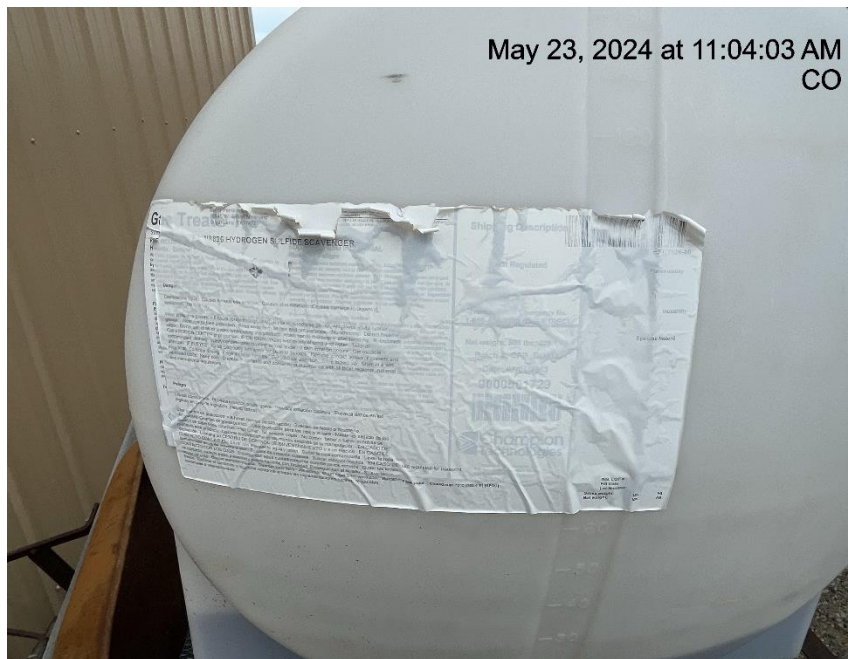
Photo # 8187 Chemical tank label weathered & damaged /illegible/does not comply with CECMC rules
