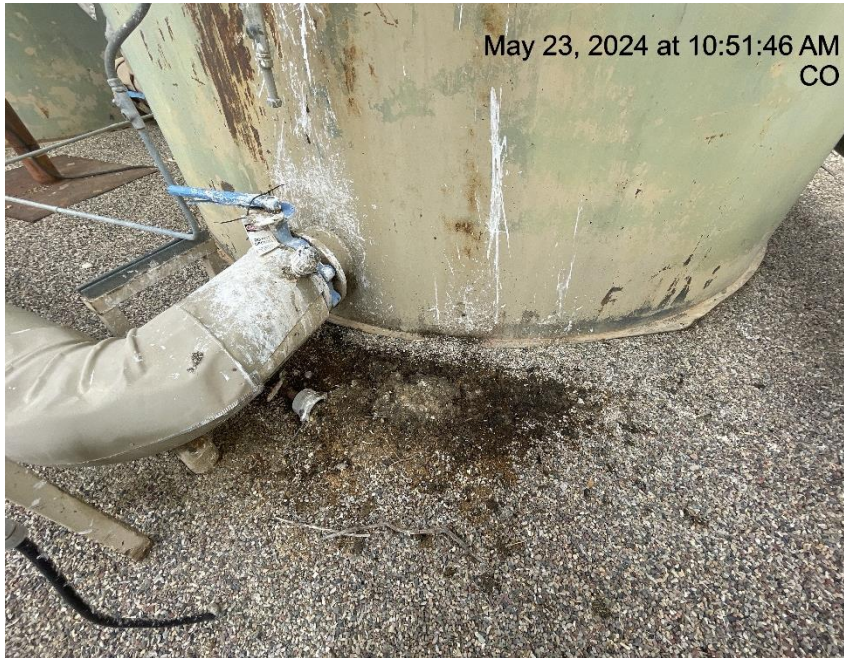
Photo # 8199 Staining in secondary containment
