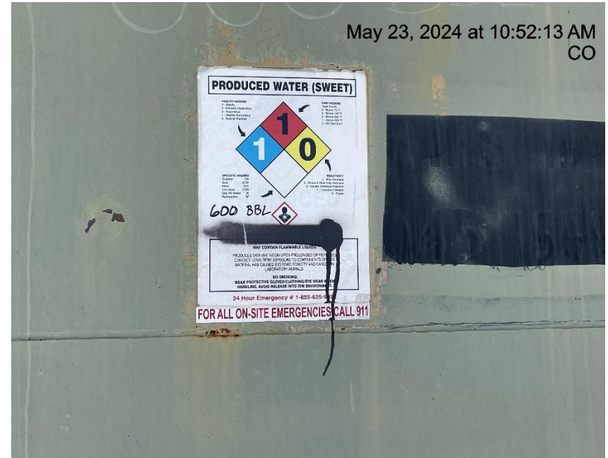
Photo # 8190 Tank label missing required information & has inaccurate information/does not comply with CECMC rules
