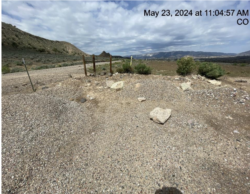
Photo # 8204 Stockpiled soils with no BMP's (S/SW corner)
