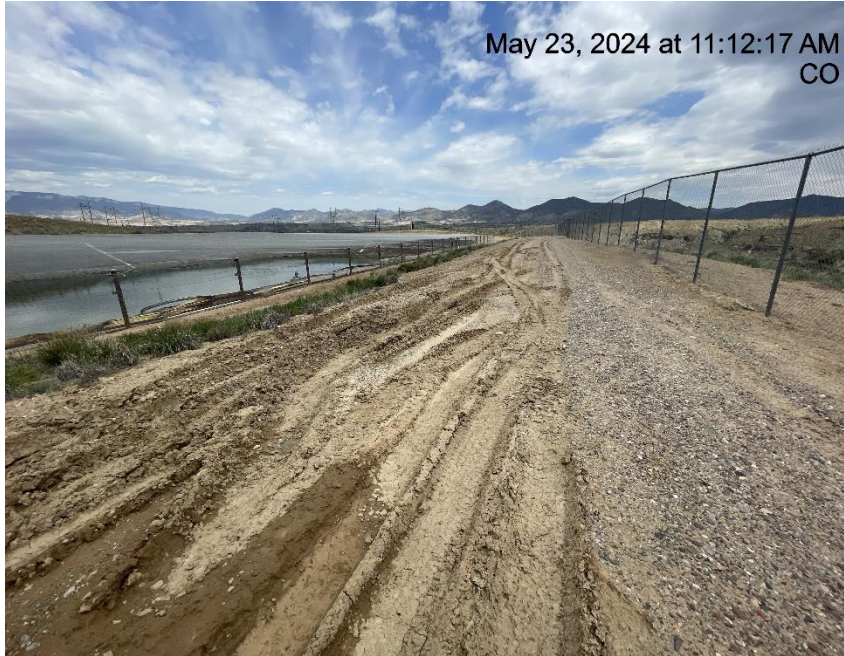
Photo # 8208 Lack of stabilization/compaction
