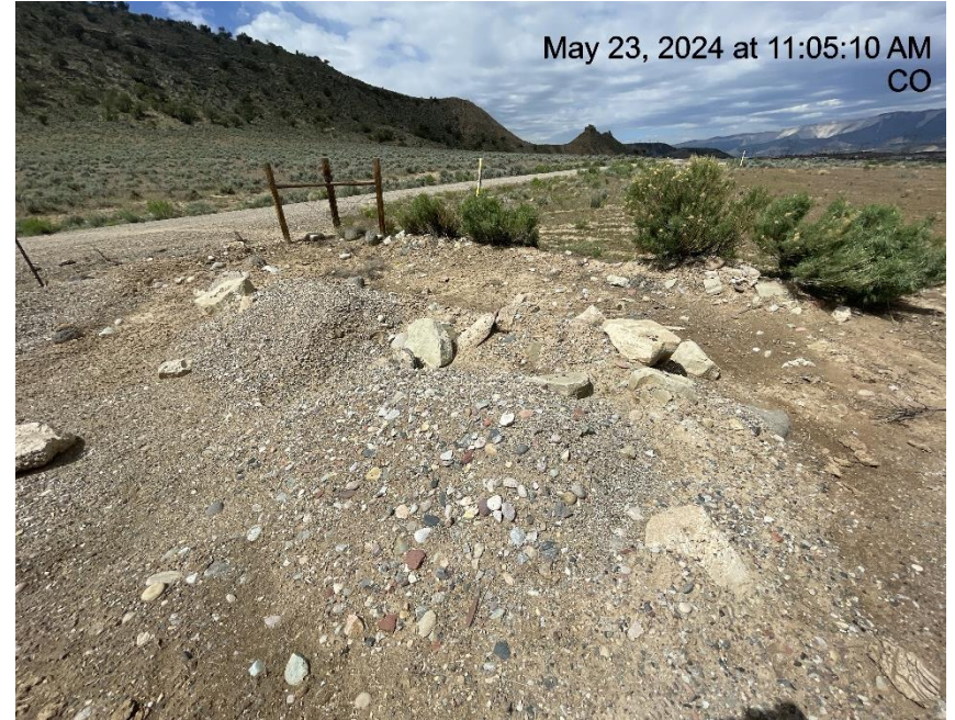
Photo # 8205 Stockpiled soils with no BMP's (S/SW corner)
