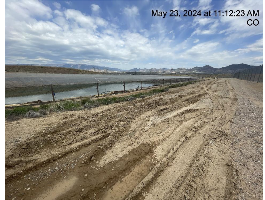
Photo # 8209 Lack of stabilization/compaction
