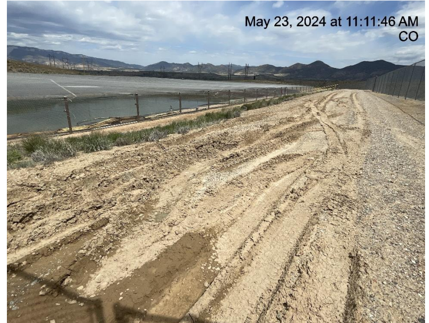
Photo # 8207 Lack of stabilization/compaction
