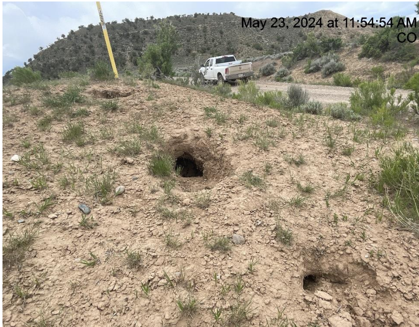
Photo # 8317 Tunnel erosion
