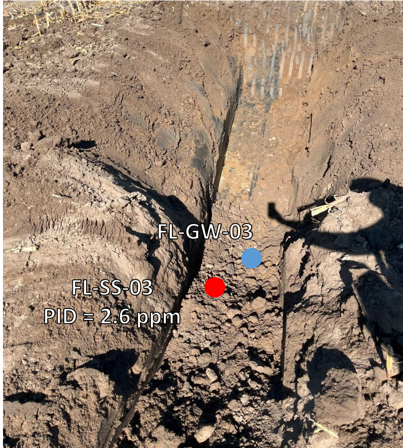
Looking north at bell hole/cut point for removal
