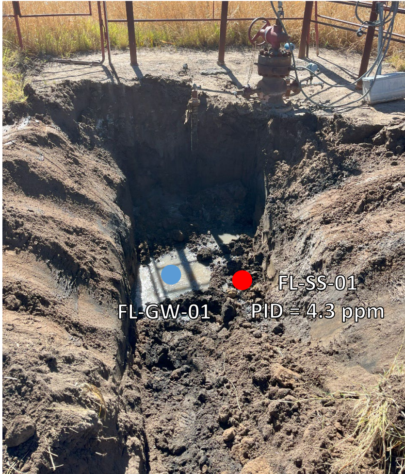
Looking south at flowline terminus/Pt. A
