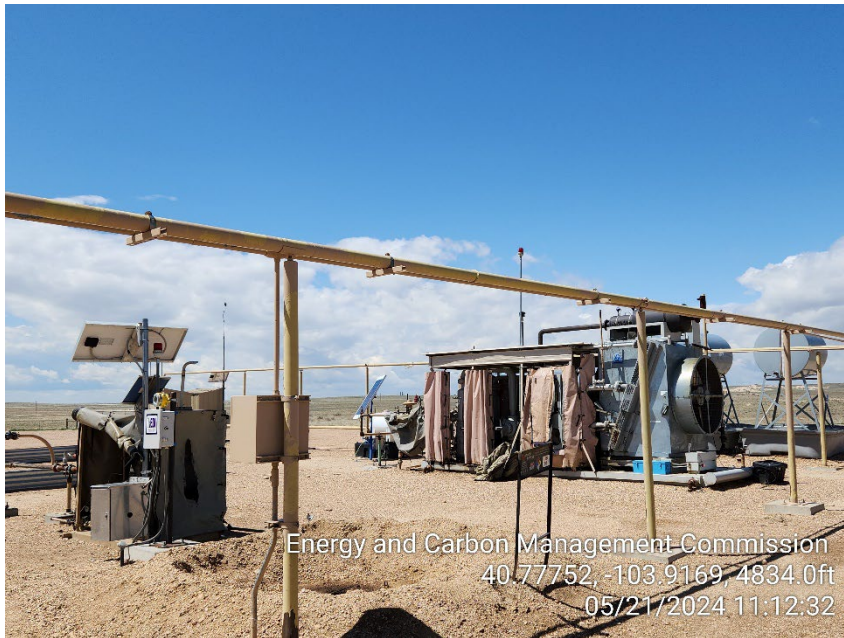
Photo 5 – VRU and Compressor
