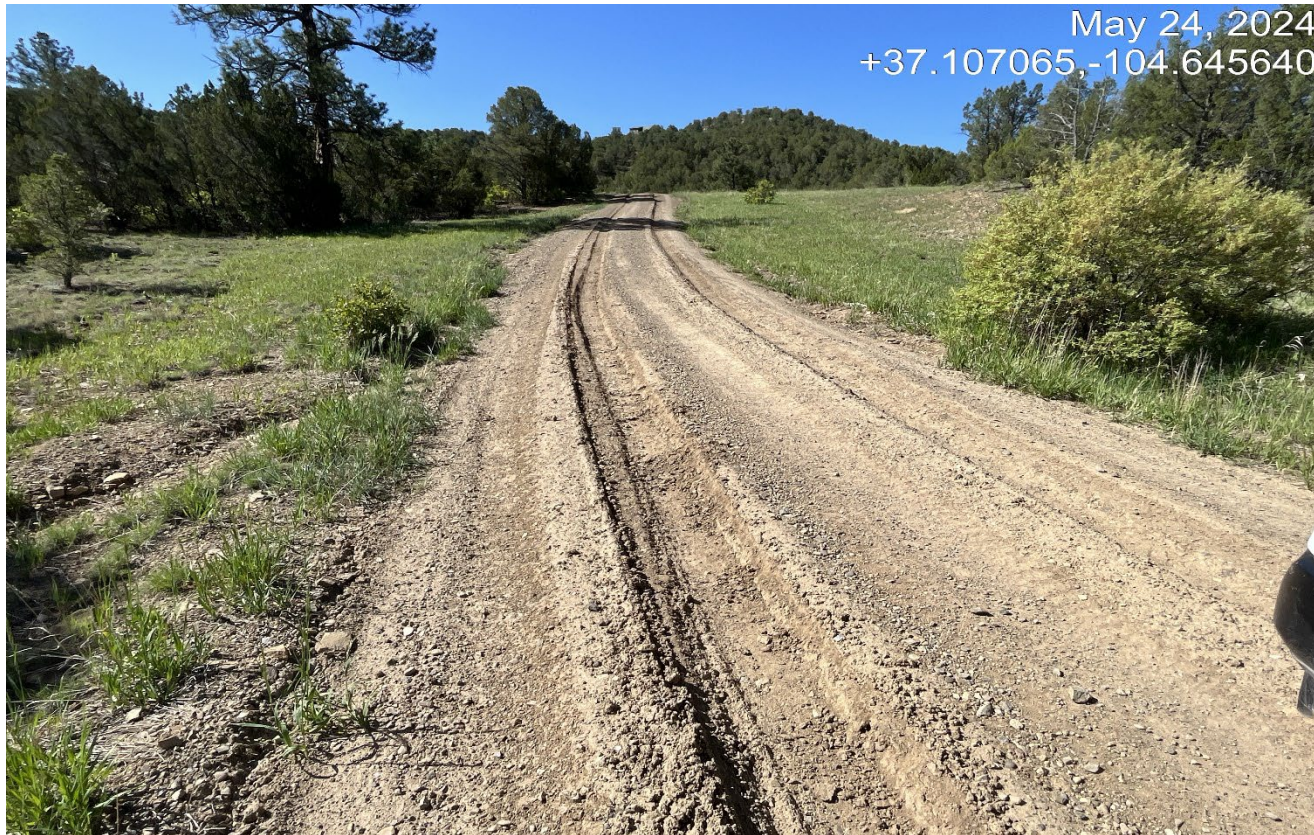
Photo 2. Facing southwest along the access road. There is vehicle rutting along the road which may need more gravel for stabilization.
