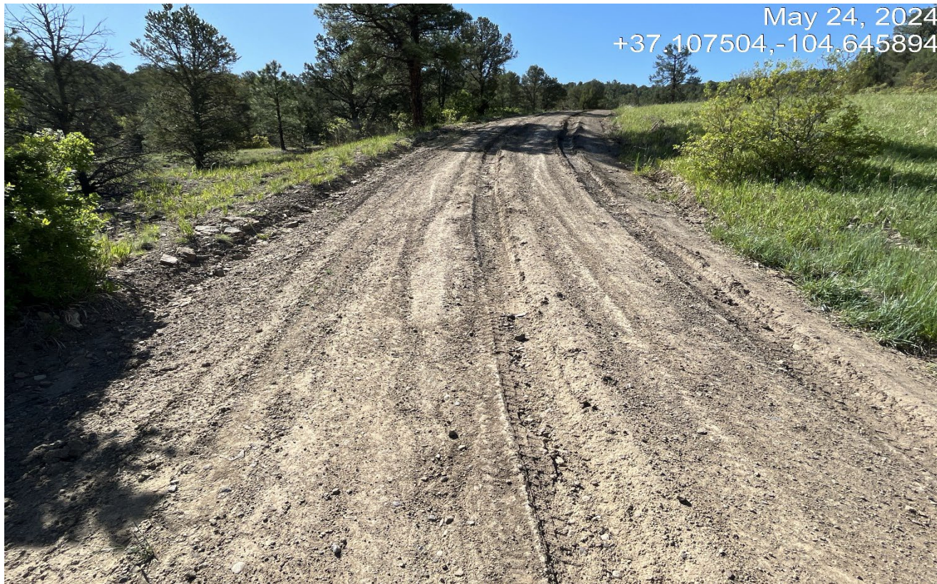
Photo 1. Facing southwest along the access road. There is vehicle rutting along the road which may need more gravel for stabilization.
