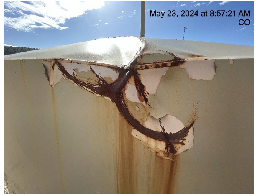
Photo # 8102 Production tank damaged
