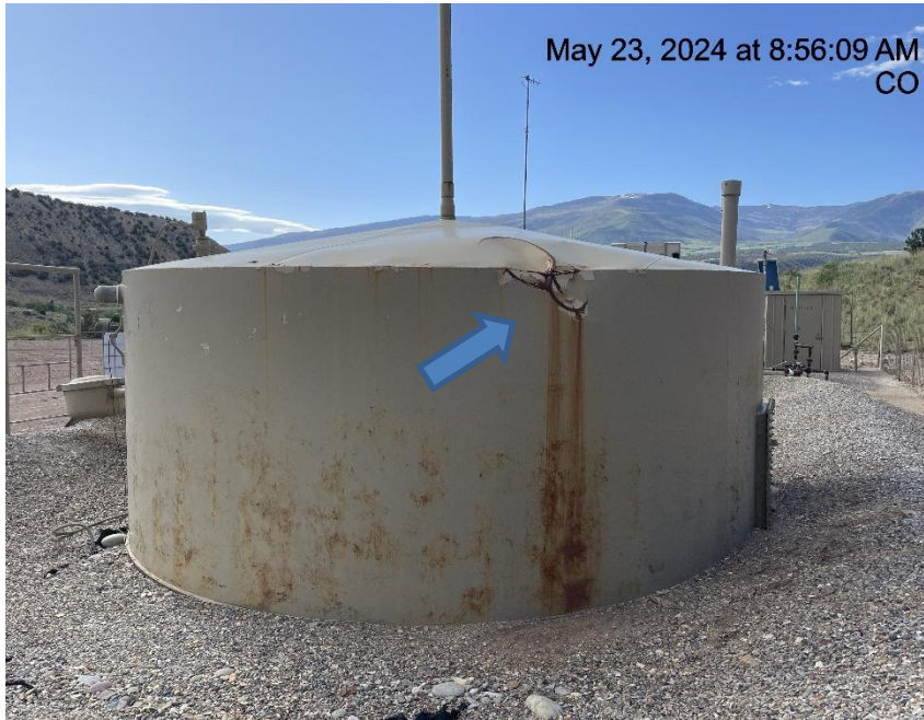
Photo # 8101 Production tank damaged
