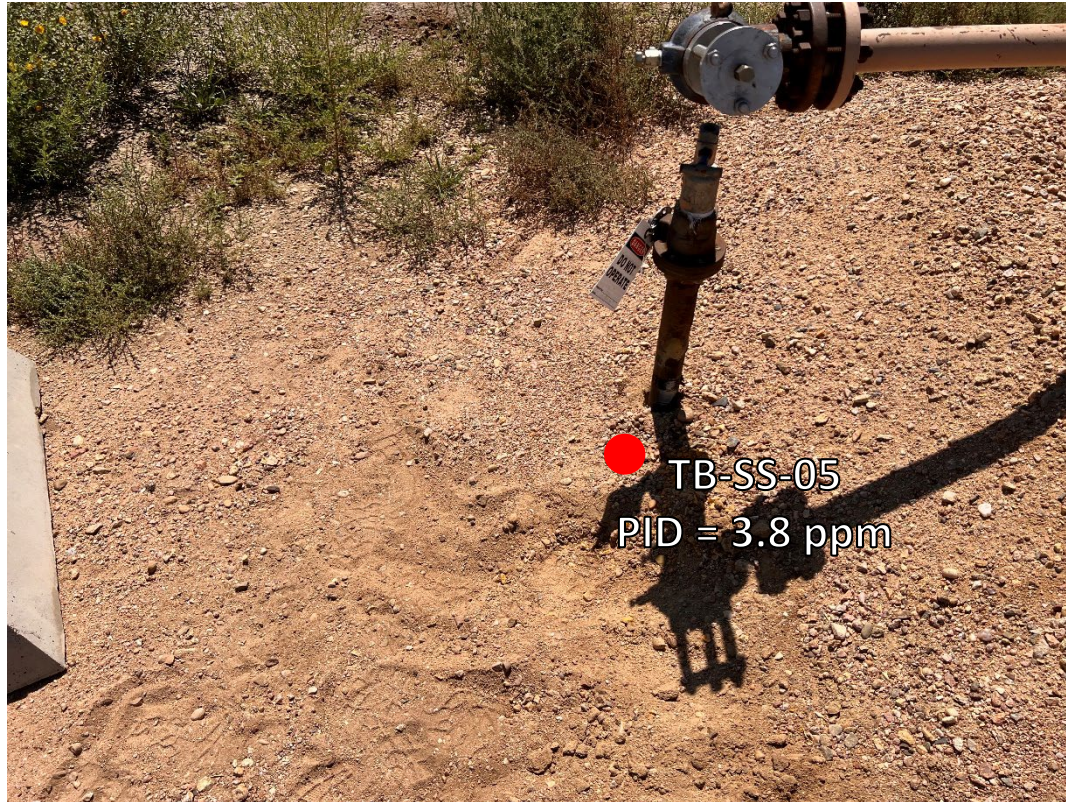
Looking south at former meter house connection
