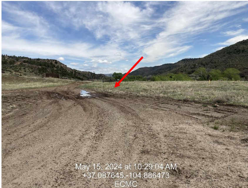
Photo 5 – Vehicle rutting
