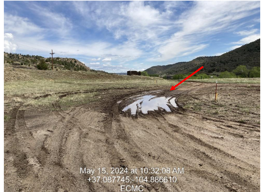
Photo 10 – Vehicle rutting
