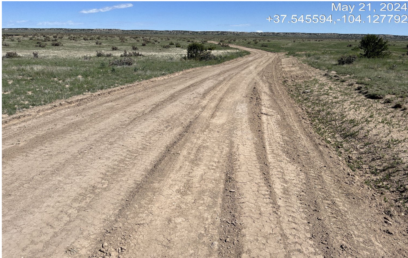
Photo 1. Facing north along the access road. The road has been regraded and crowned.
