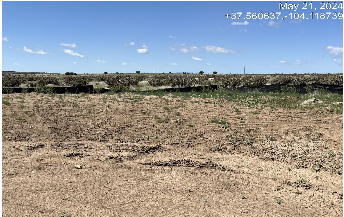
Photo 7. There are several areas where the silt fence is not maintained.
