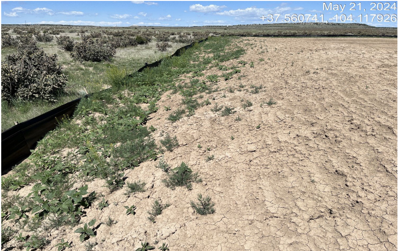
Photo 6. Facing toward the soil stock pile. There weeds beginning to grow along the soil pile. The topsoil must be seeded to prevent weed establishment.
