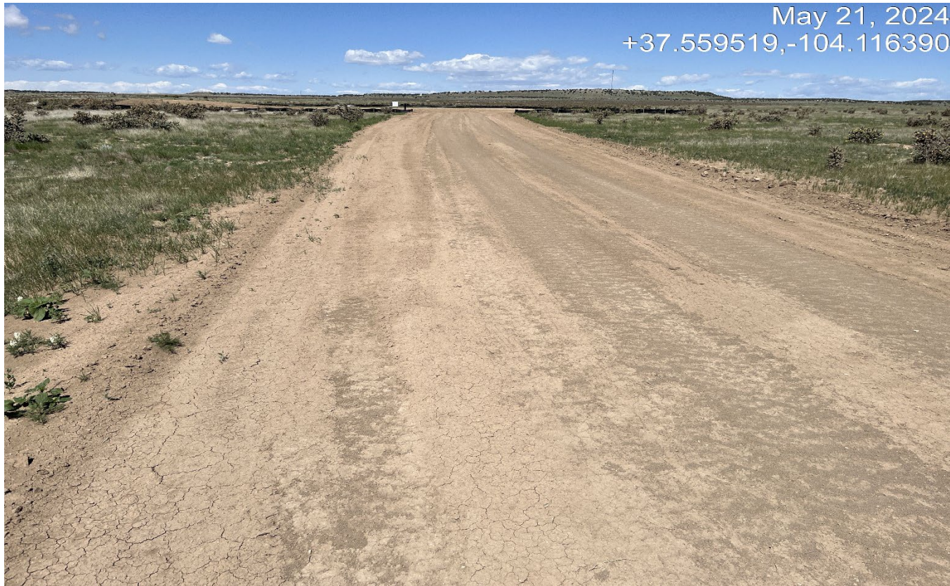
Photo 3. Facing northwest toward the access road. The side of the road needs to be seeded and stabilized.
