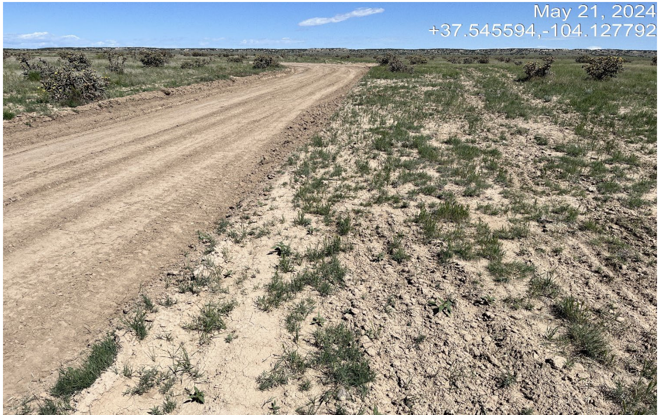
Photo 2. Facing north along the road. The vehicle ruts outside of the road have been raked out.
