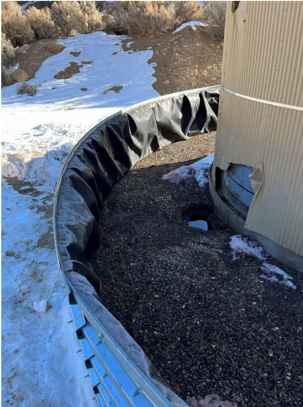
12/14/2023 – Photo showing containment following free liquid removal
