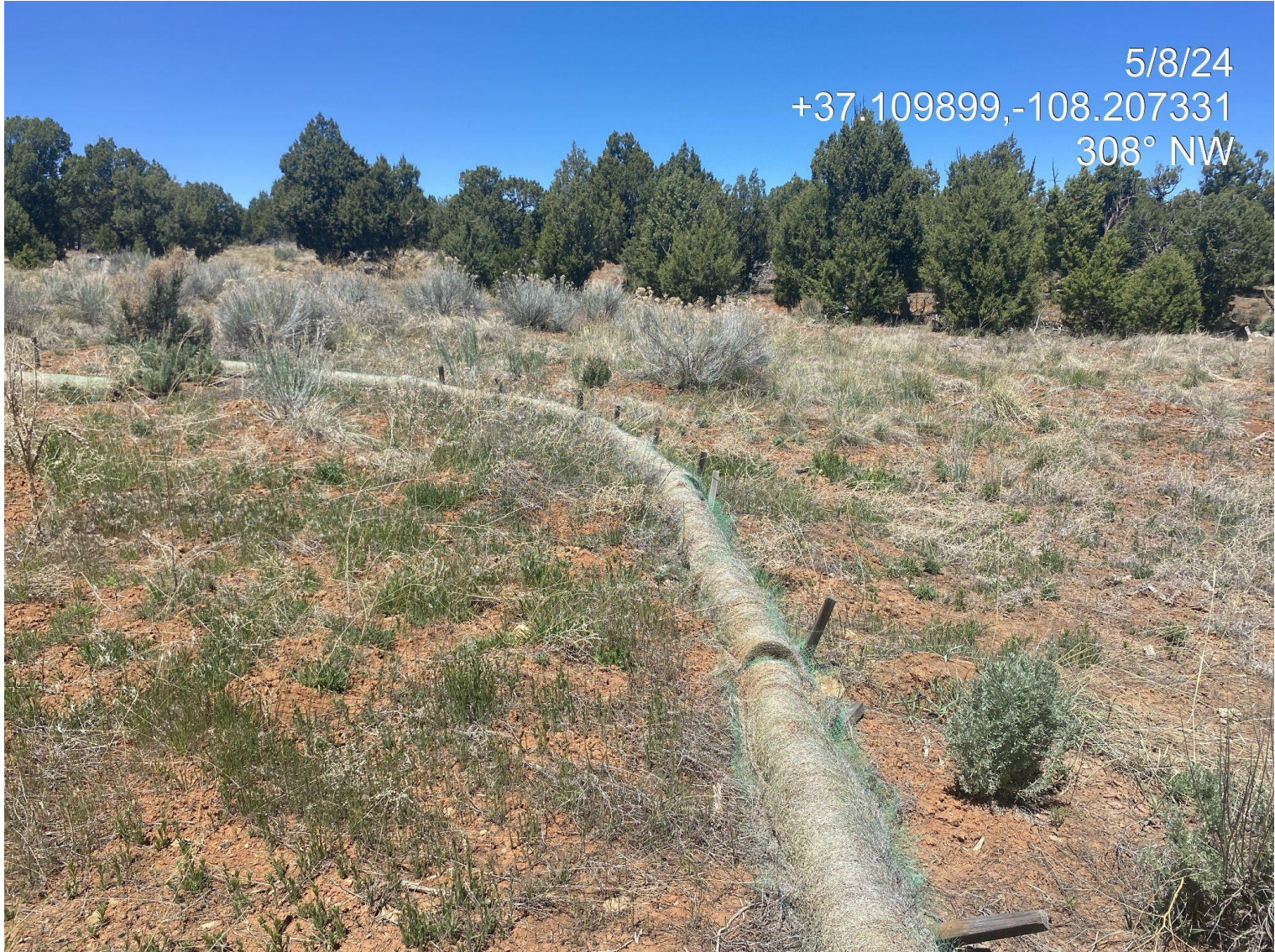
Photo 5. View of straw wattles that remain on location.
