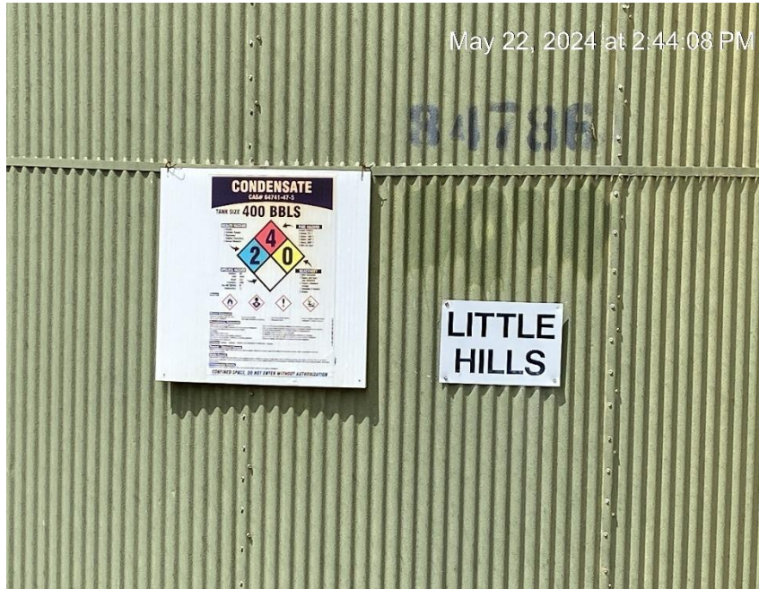
Tank labeling missing required information
