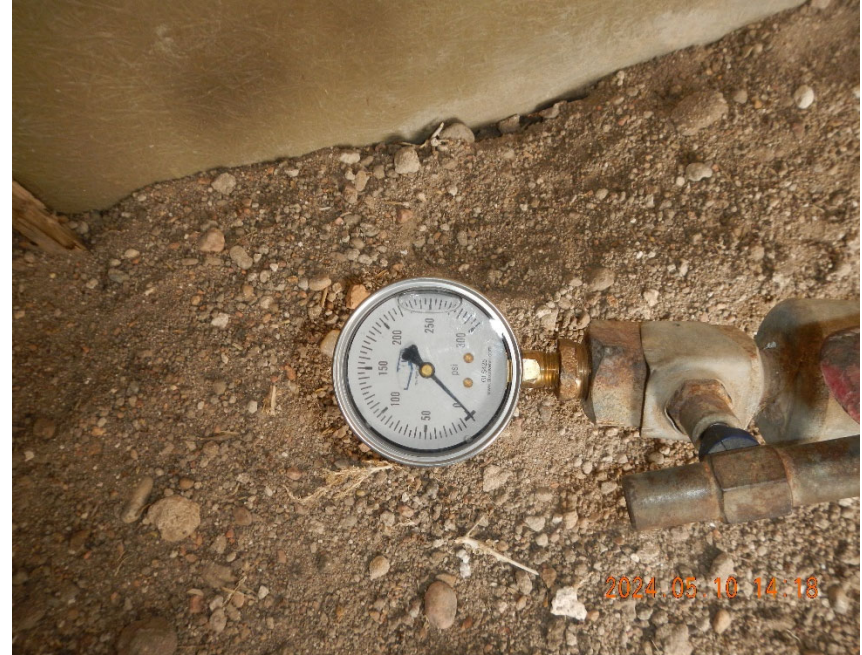
4. Casing pressure at time of inspection.
