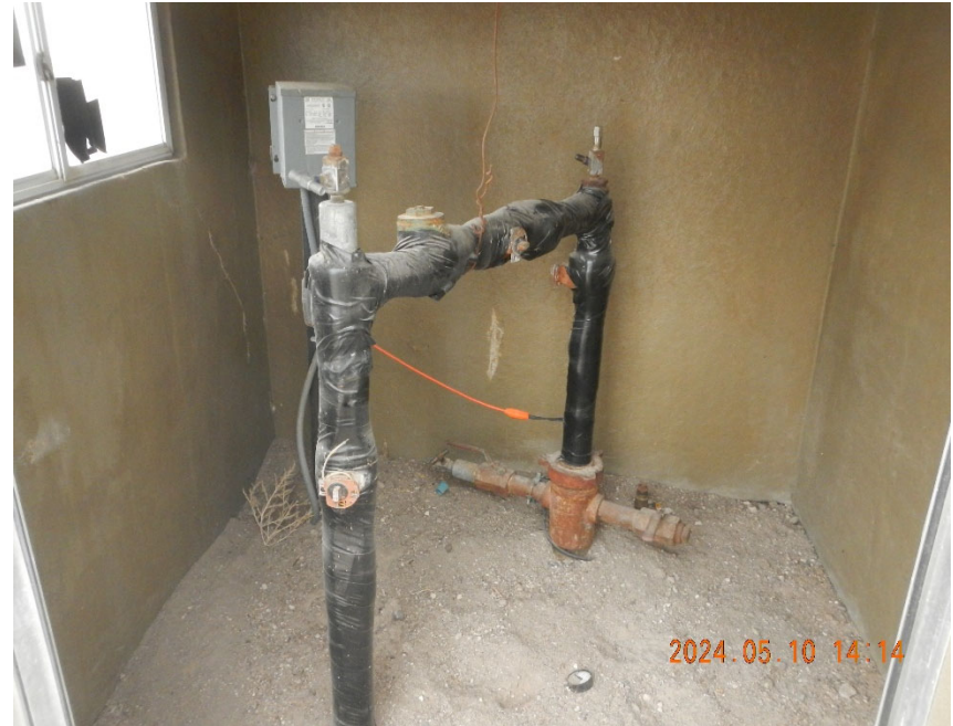
2. View f wellhead.
