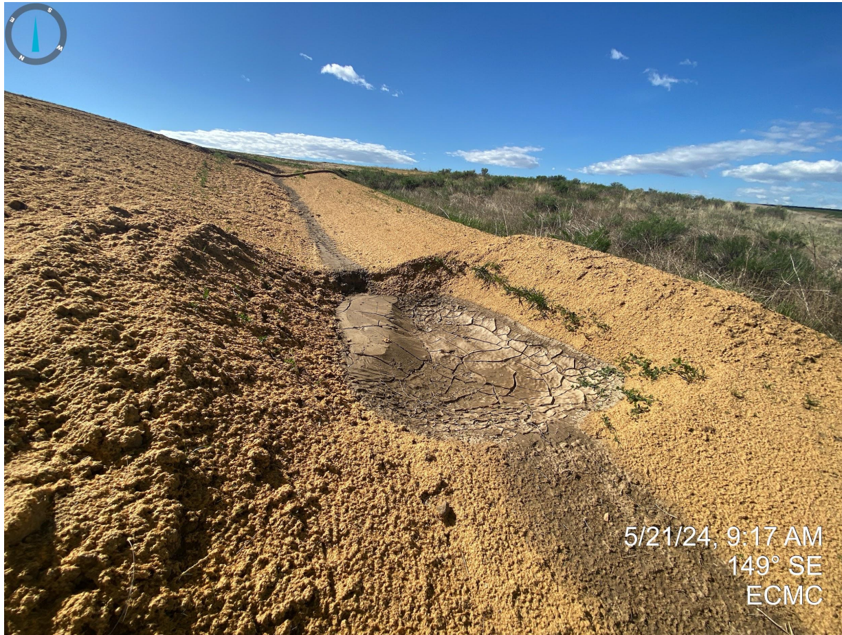
Photo 17. Sediment trap requires maintenance.
