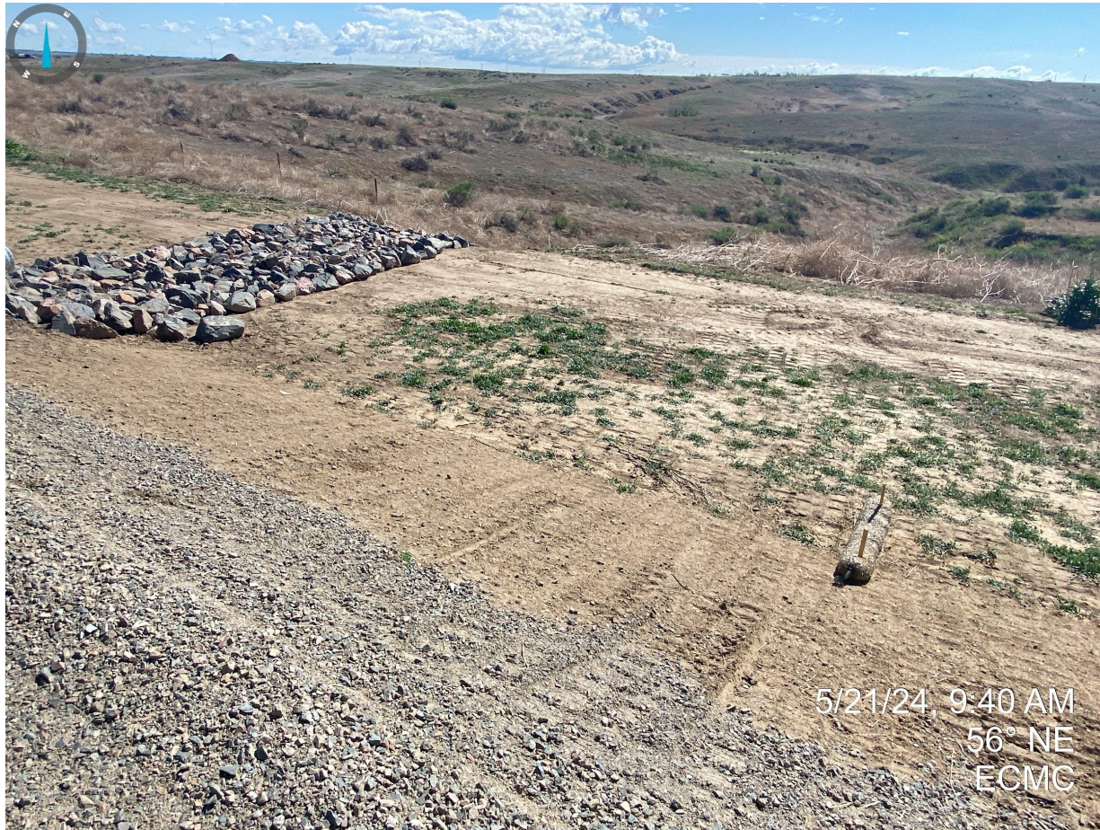
Photo 2. Erosion degradation previously documented appears to have been repaired and stormwater control measures/BMPs have been installed.
