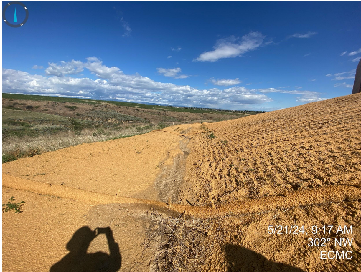
Photo 16. Erosion degradation (e.g. riling and sediment deposition) observed on the west portion of the location. BMPs require maintenance.
