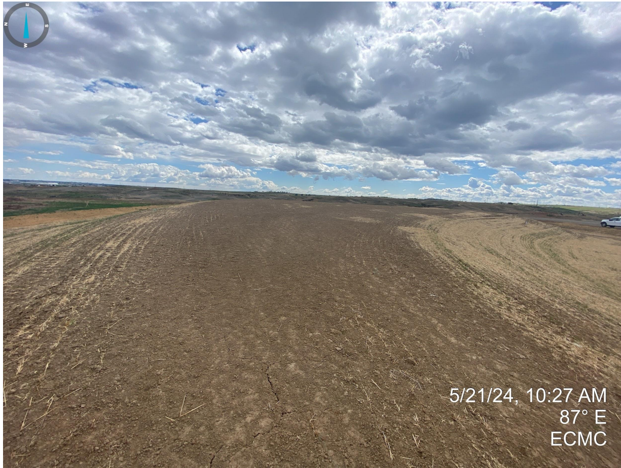
Photo 9. Taken from the top/upper portion of the topsoil stockpile. Photo illustrates that straw mulch appears to have blown off the top, though, germination was evident. Operator will need to monitor and manage the stockpile to ensure that it is properly protected against wind/water erosion and stabilized for long term until interim reclamation commences.
