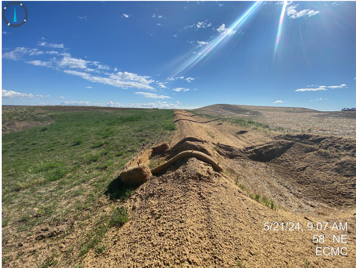
Photo 10. Taken from the north/northwest portion of the disturbance area. Perimeter ditch and berm soils appear to have been stabilized with hydromulch.
