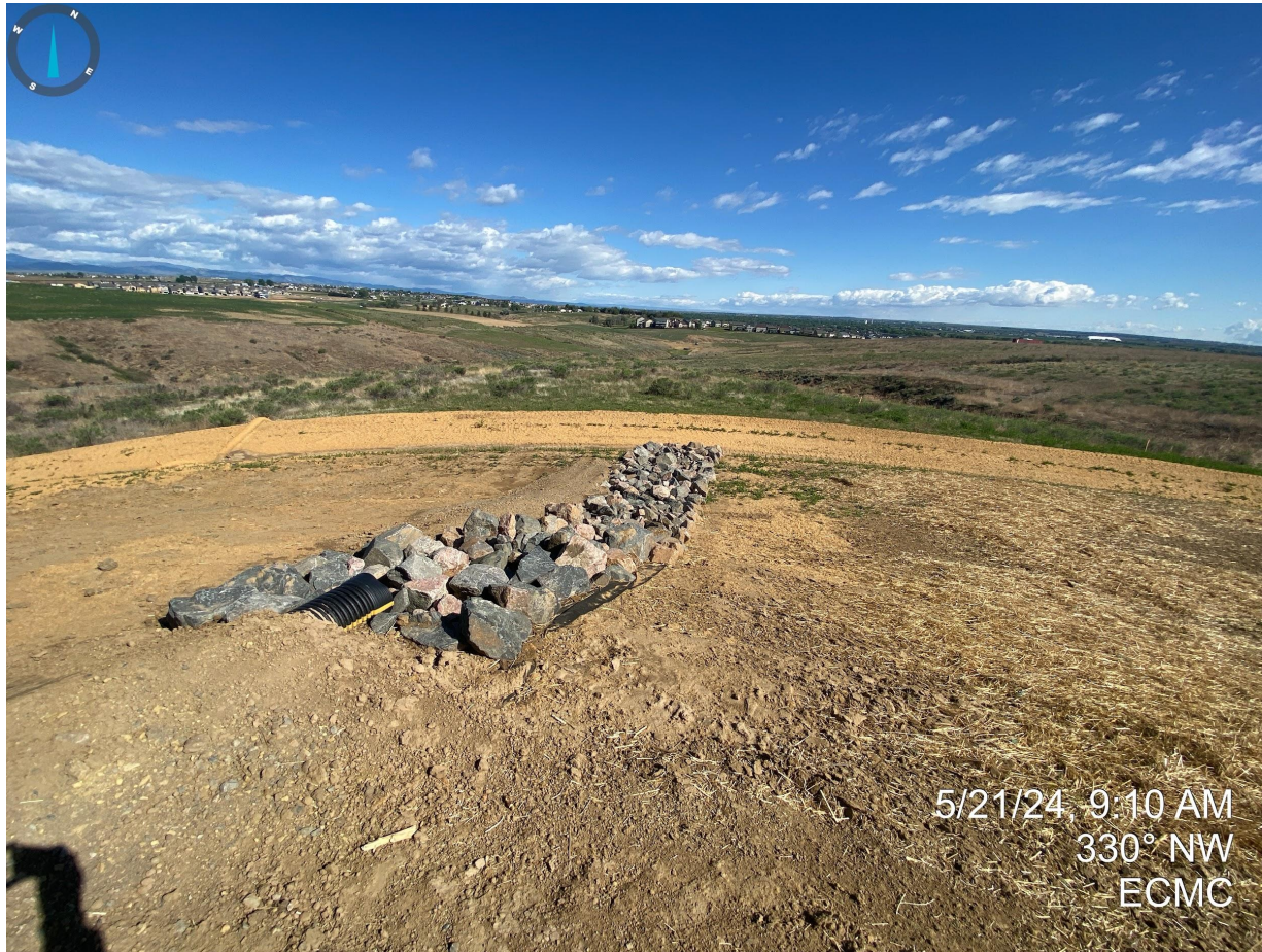
Photo 12. Armored spillway located on the northwest corner of the drilling pad.
