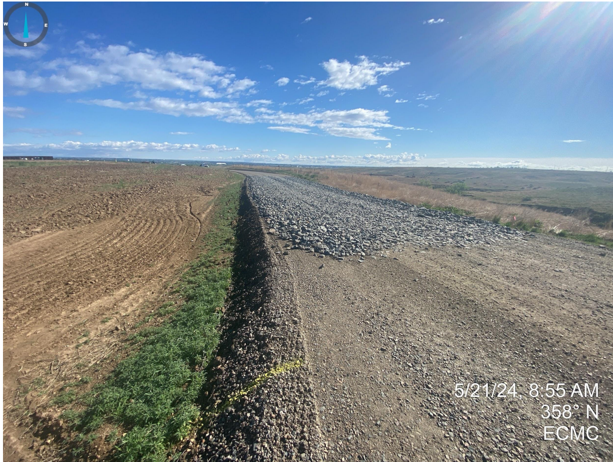
Photo 1. Track Out pad installed at the access road entrance.
