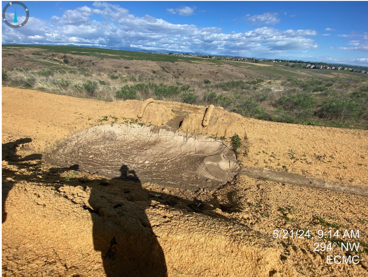
Photo 15. Sediment trap requires maintenance.
