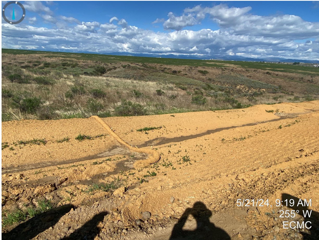
Photo 18. Erosion degradation (e.g. riling and sediment deposition) observed on the west portion of the location. BMPs require maintenance.
