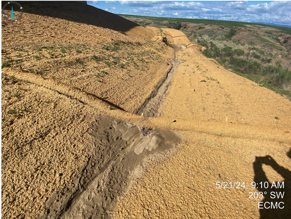
Photo 13. Erosion degradation (e.g. riling and sediment deposition) observed on the northwest portion of the location. BMPs require maintenance.
