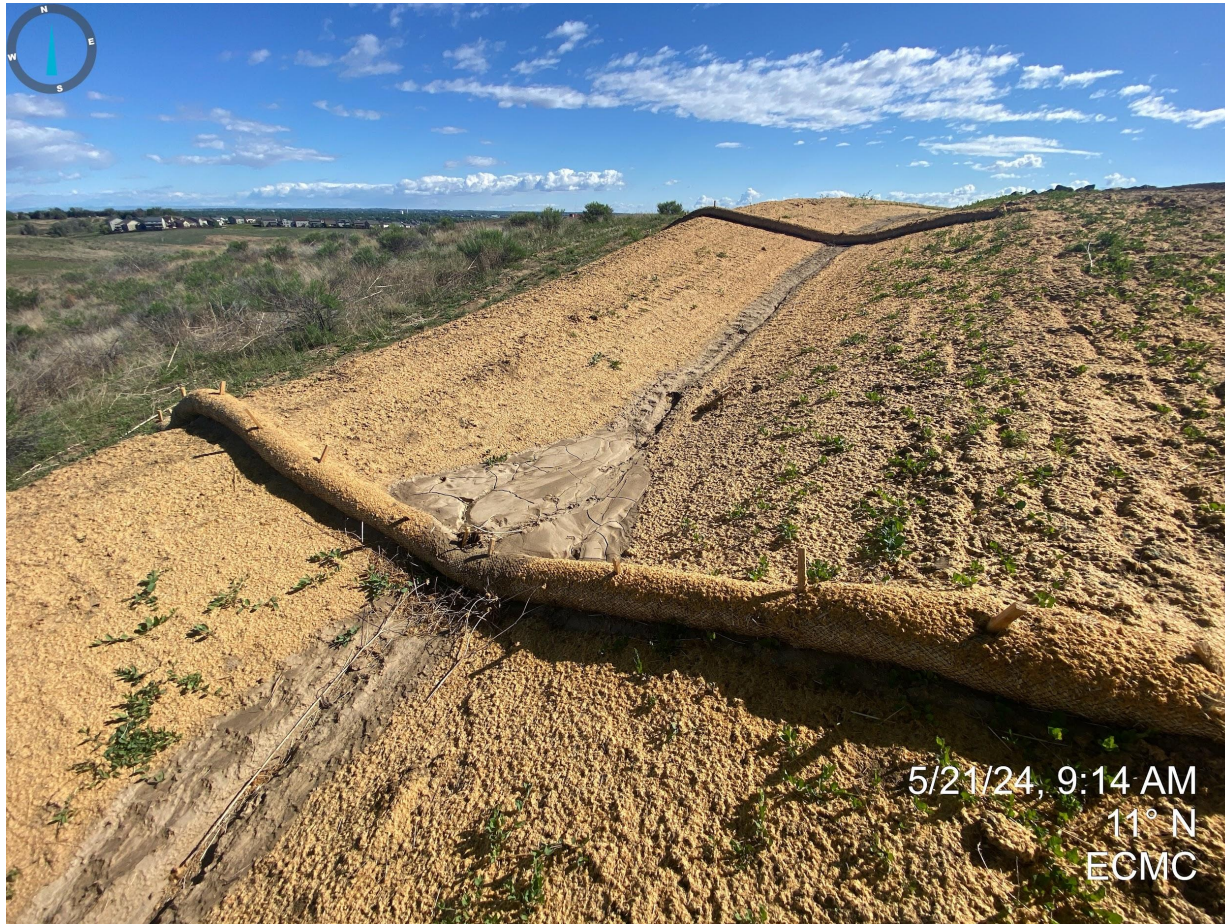
Photo 14. Erosion degradation (e.g. riling and sediment deposition) observed on the northwest portion of the location. BMPs require maintenance.
