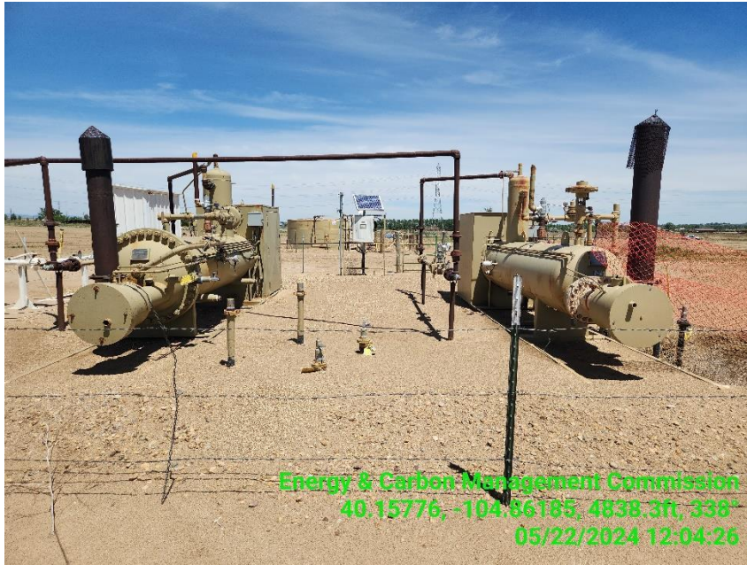
Photo 5 Horizontal Heated Separators, LOTO.
